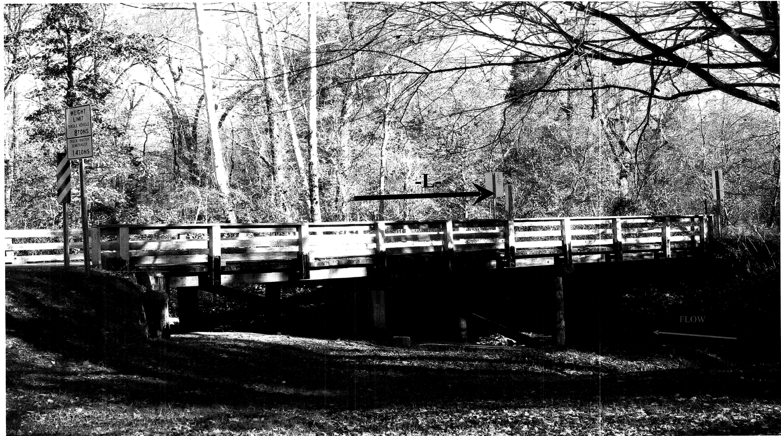
Looking Northeast towards End Bent 2
