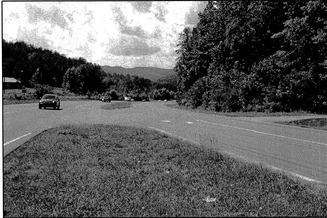
PHOTO TAKEN ALONG INTERIOR BENT LOOKING RIGHT.
