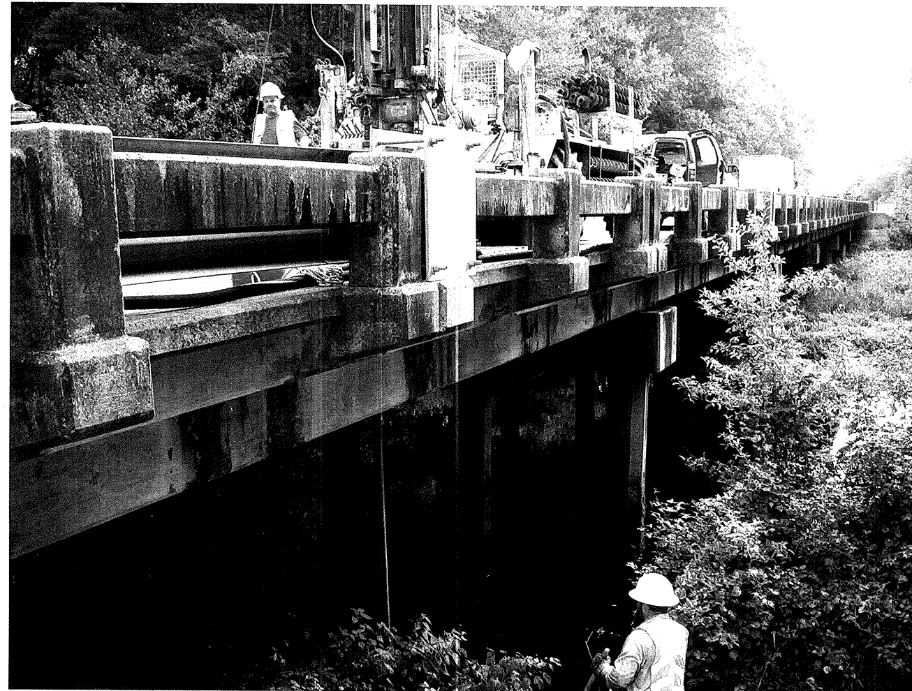
View facing East along South side of existing bridge
