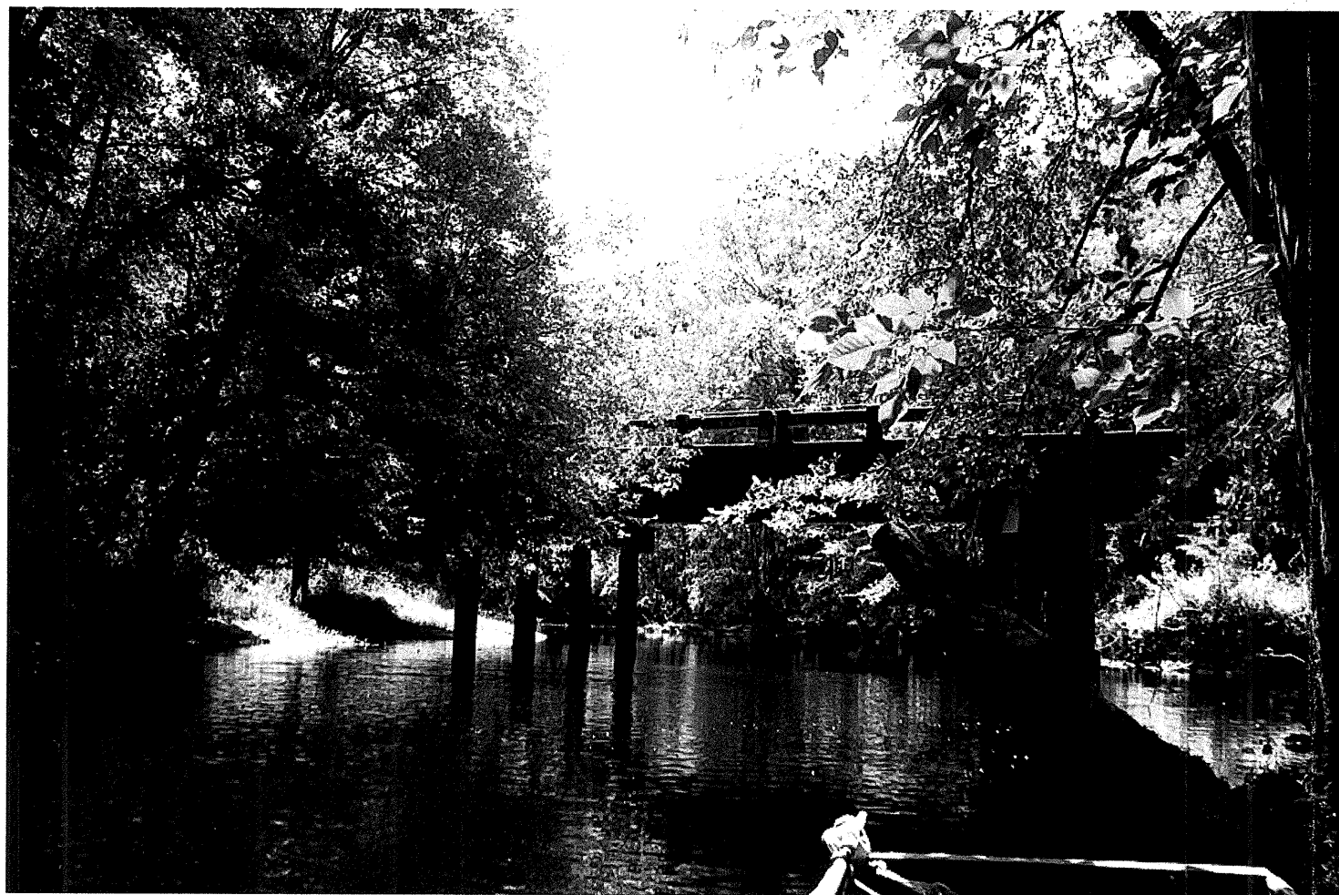
View of existing bridge facing North (upstream) from Lumber River
