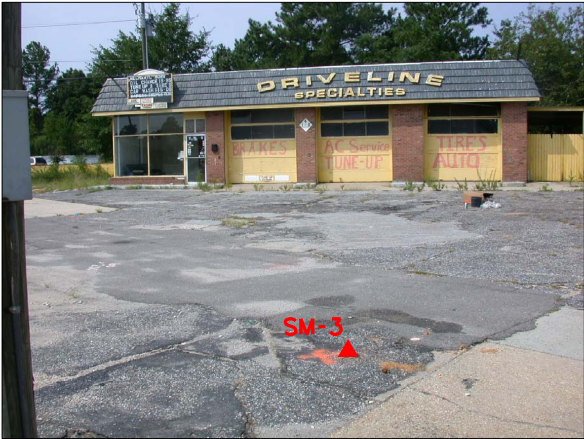
PHOTO 3 - BORING WITHIN PROPOSED R/W LOOKING WEST
