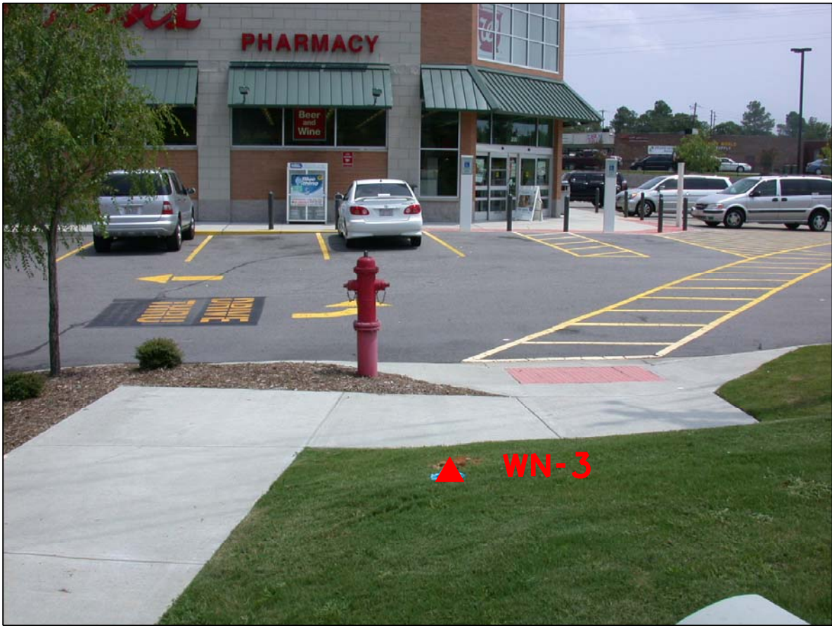
PHOTO 3 - BORING WITHIN PROPOSED R/W LOOKING EAST
