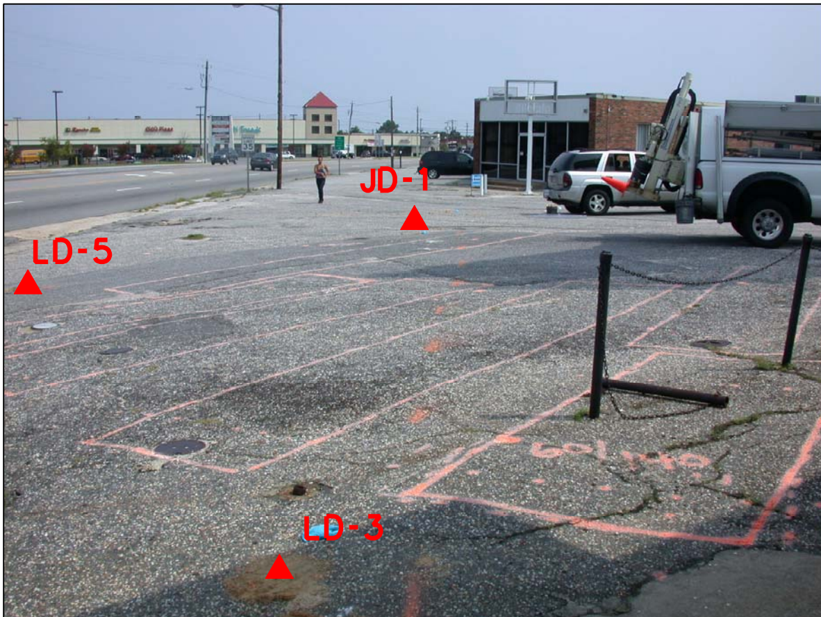
PHOTO 6 - BORINGS WITHIN PROPOSED R/W LOOKING NORTHEAST ALONG R/W
