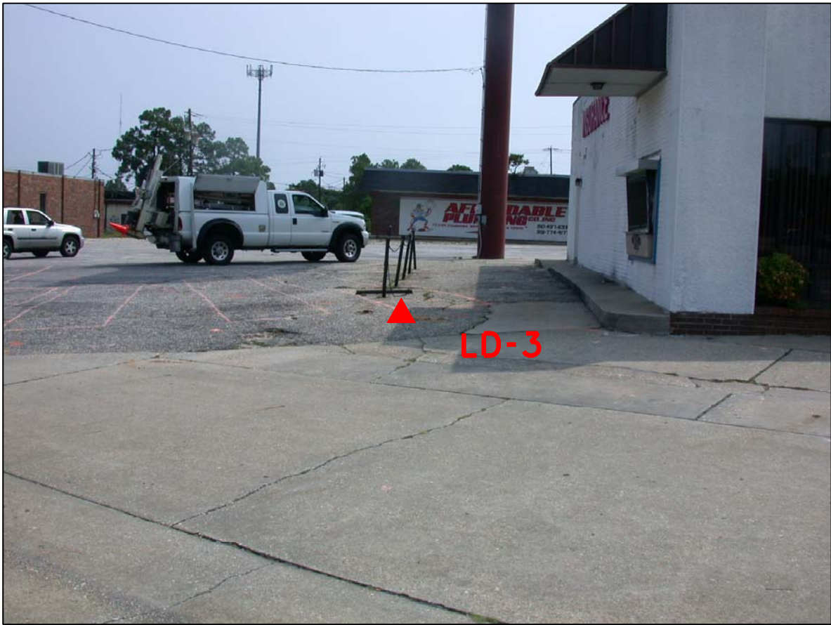
PHOTO 3 - BORING WITHIN PROPOSED R/W LOOKING EAST
