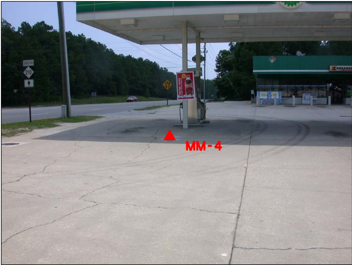
PHOTO 3 - BORING WITHIN PROPOSED R/W LOOKING SOUTHEAST
