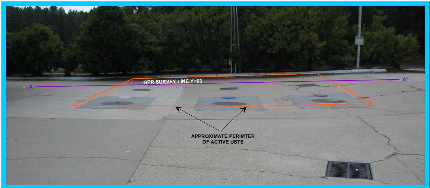
The orange rectangle in the photograph represents the approximate perimeter of the three active metallic USTs, as suggested by the GPR data, centered near grid coordinates X=395 Y=60. The solid purple line in the photograph represents the approximate location of the GPR image shown above. The photograph is viewed in a southwesterly direction.
