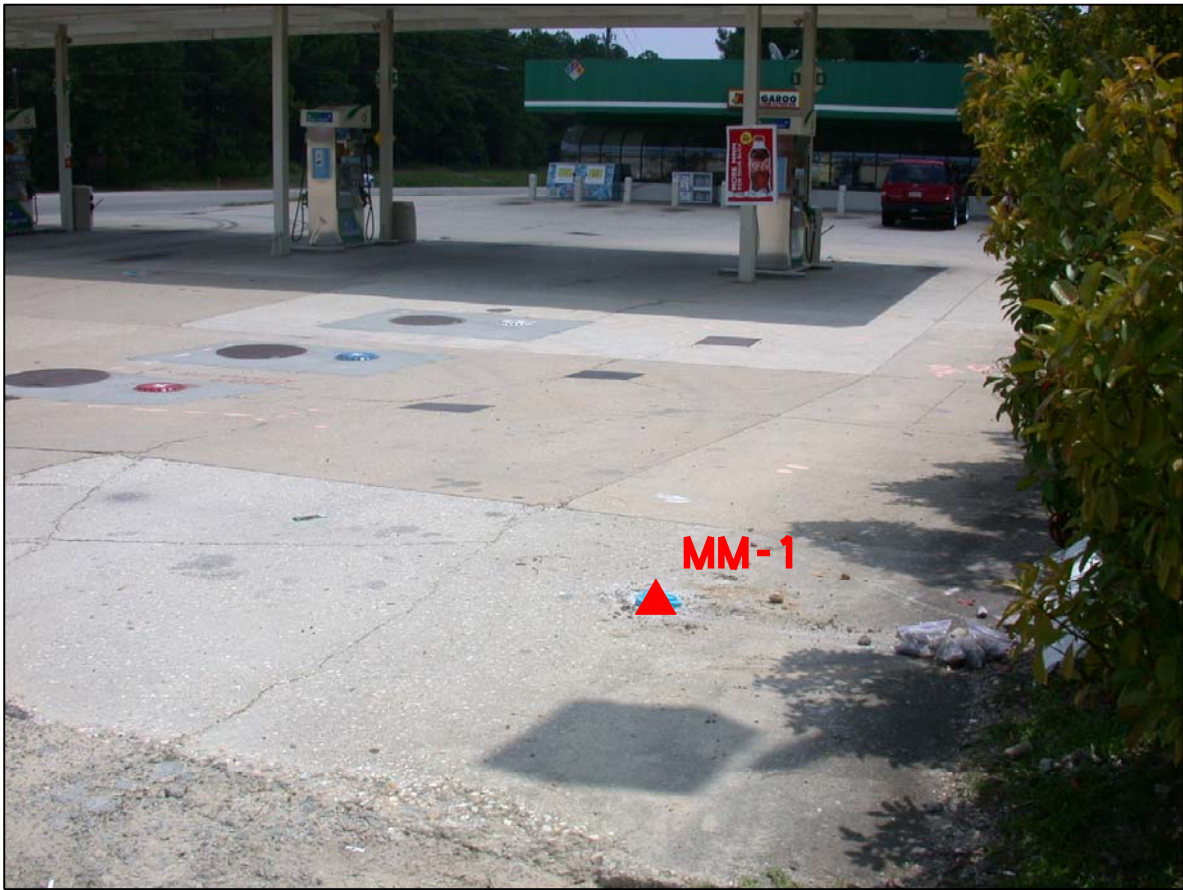
PHOTO 1 - BORING IN PROPOSED R/W LOOKING SOUTHEAST
