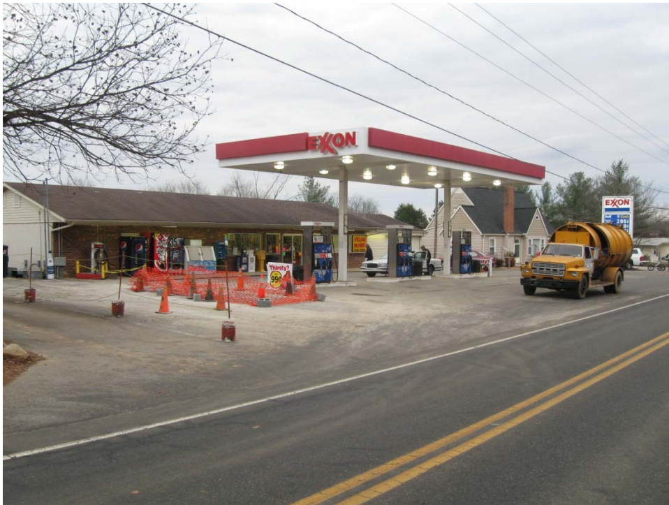
Parcel 199 – S.L. Jarvis & M.C. Jarvis Property, looking southeast
