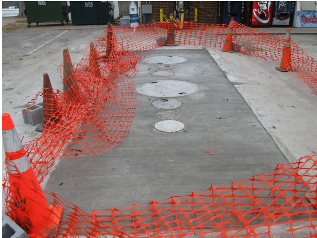
Parcel 199 – S.L. Jarvis & M.C. Jarvis Property, looking southeast. Photo shows location of new slab poured over the known UST near the north side of the property.
