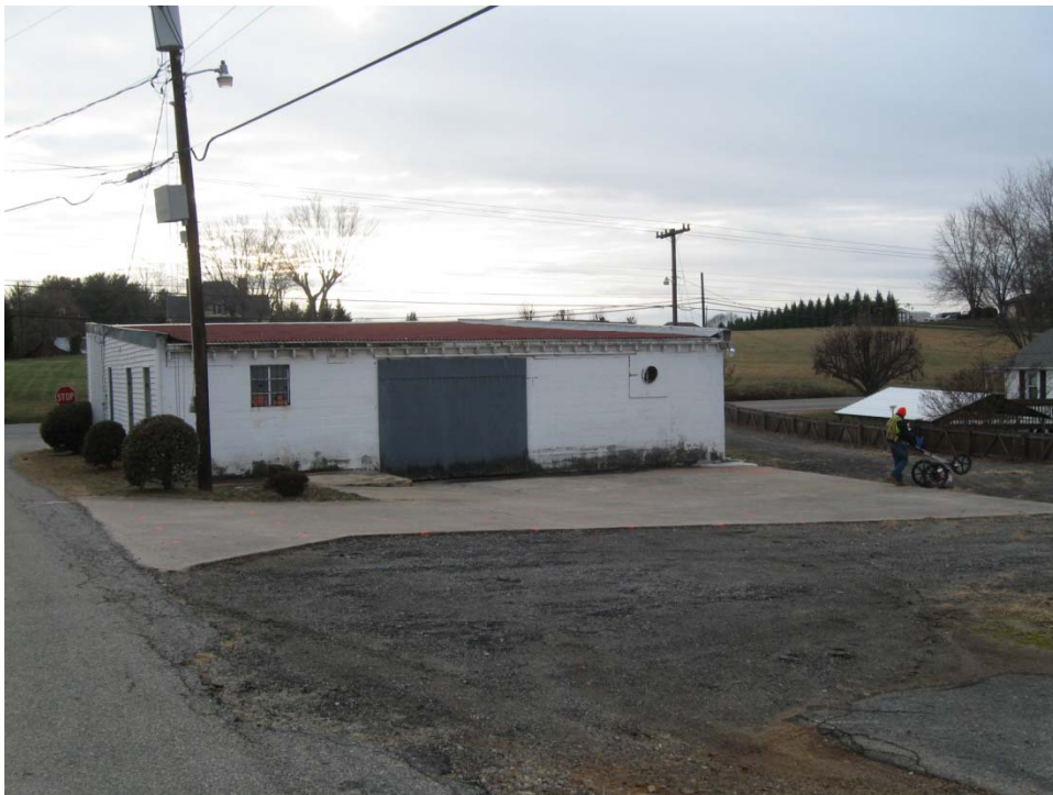
Parcel 98 – Steven Joseph Whitley Property, looking west
