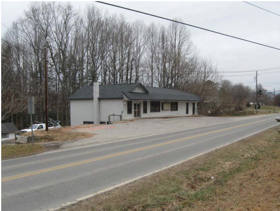
Parcel 51 – R.D. Mitchell Property, looking northwest
