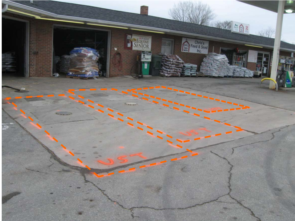
Parcel 1 – James C. Pardue Property, looking east. Photo shows approximate marked location of Known UST Nos. 1-3 on the northwest side of the canopy.
