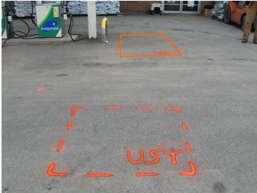
Parcel 1 – James C. Pardue Property, looking east. Photo shows approximate marked location of Probable UST Nos. 2 and 4 near the southeast edge of the canopy.
