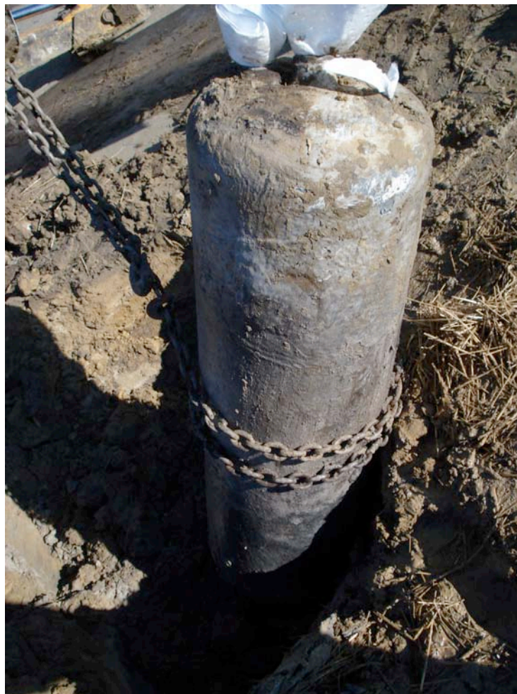
Photograph 4: View looking northwest at UST #002 during removal.
