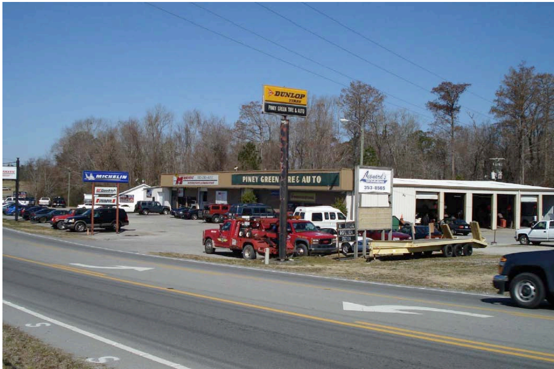
Photograph 1: View looking northwest at Parcel 149 in November 2010 when facility was in operation.
