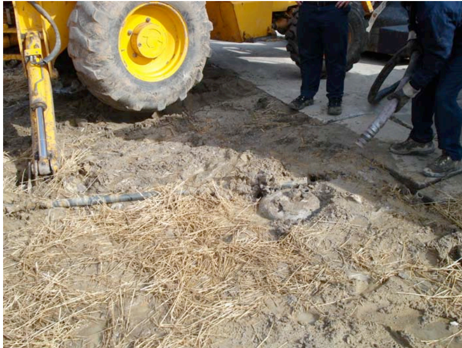
Photograph 3: View looking northeast at UST #001 prior to removal.
