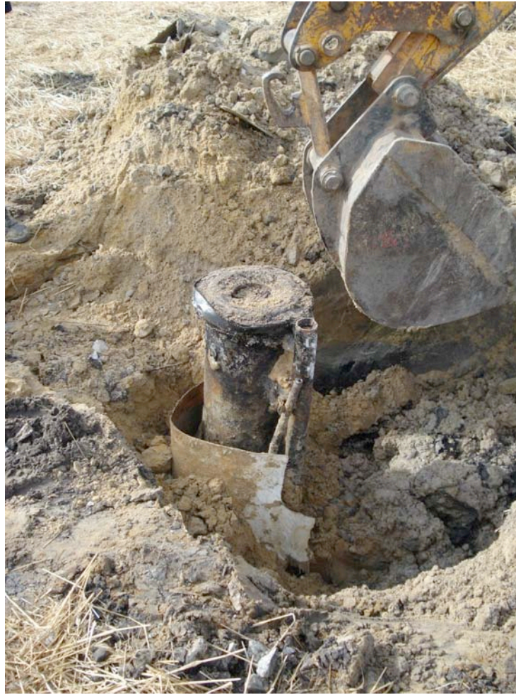
Photograph 7: View looking northwest at Lift 3 during removal. Sidewalls show stained soil.
