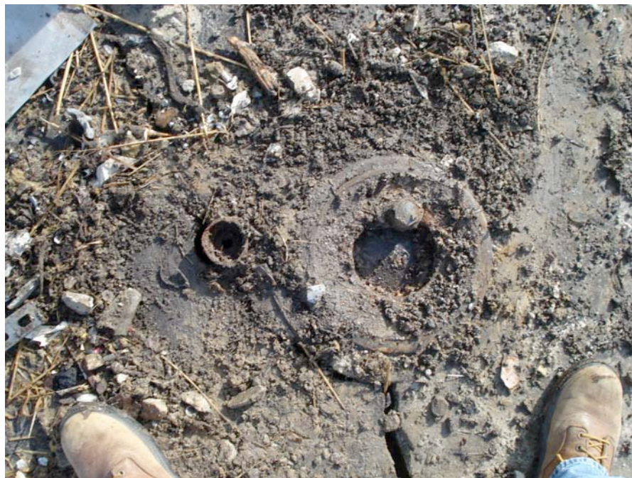
Photograph 6: View looking down at Lift 3 prior to removal.
