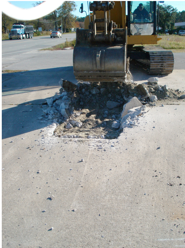
Photograph 1: View looking south at beginning of excavation across "Possible USTs" area.
