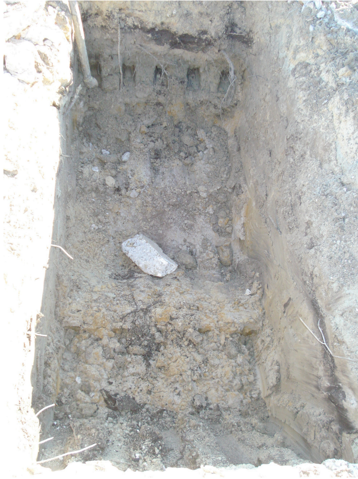
Photograph 3: View looking south at completed excavation.
