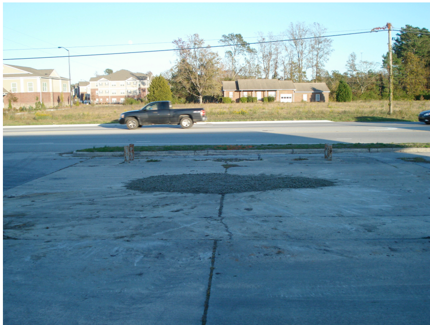
Photograph 4: View looking east at backfilled and compacted excavation.
