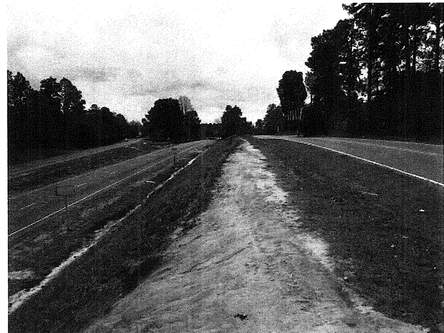
Photo No. 4: Wall 2 – along top of slope looking southwest
