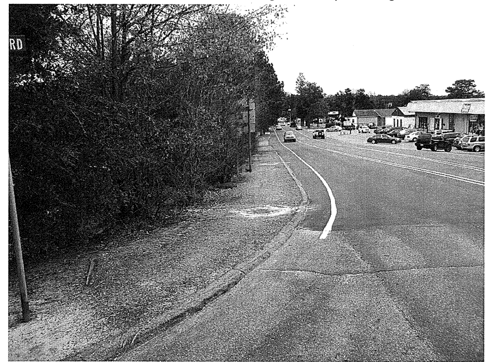
Photo No. 2: Wall 3 – along top of slope looking southeast
