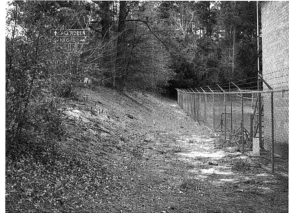
Photo No. 1: Wall 3 – along toe of slope looking northwest
