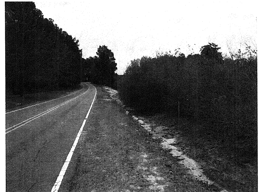
Photo No. 2: Wall 2 – along top of slope looking northeast
