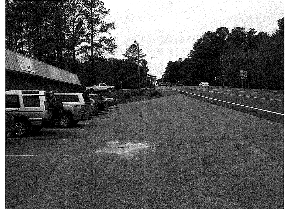
Photo No. 1: Wall 4 – along wall looking northwest
