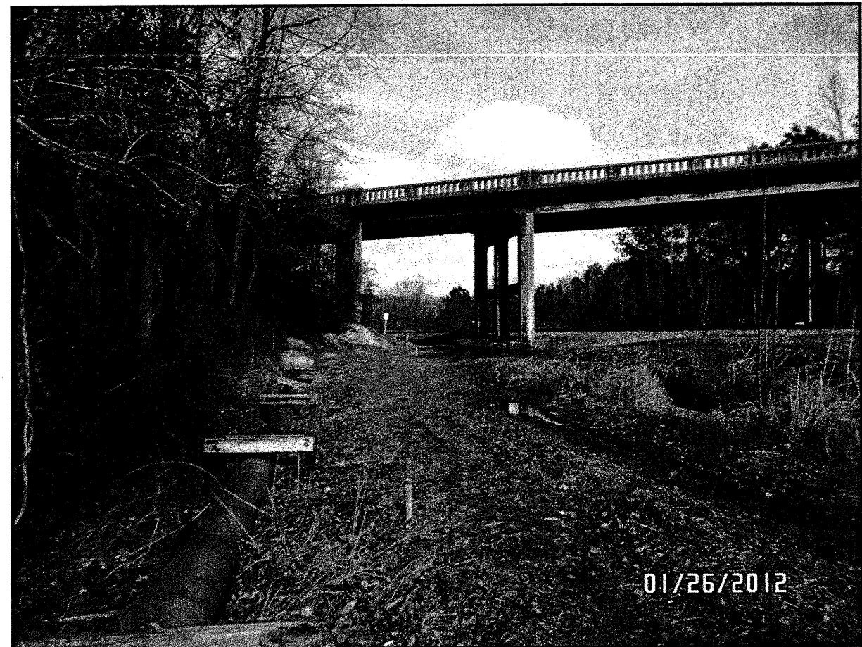
BENT 1, LOOKING FROM RT TO LT.
