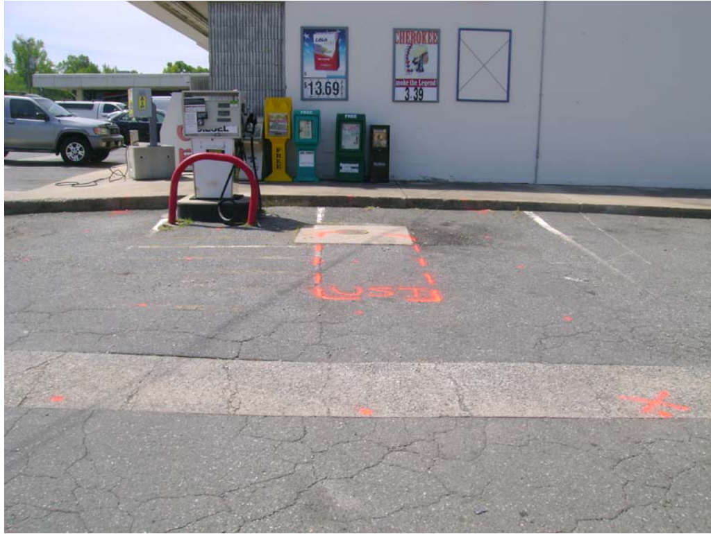
Parcel 110 – Ilesh & Hema Shah Property, looking south. Photo shows approximate marked location of the known UST near the northeastern building corner.
