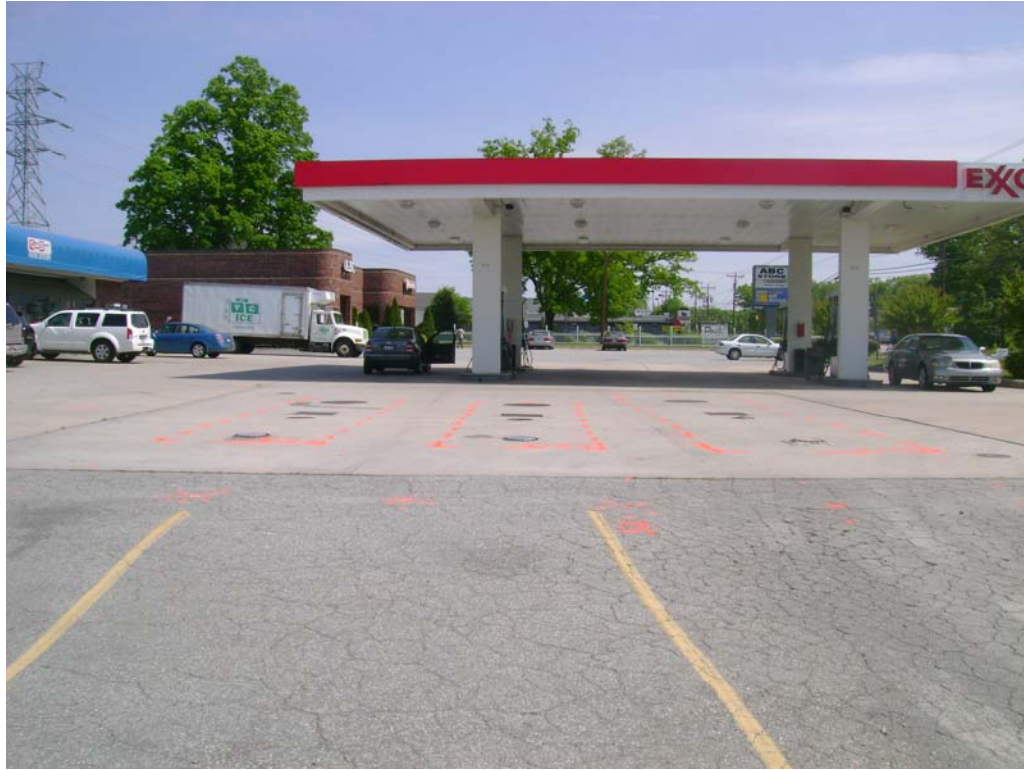
Parcel 32 – C. Richard Bruning IV Property, looking northeast. Photo shows approximate marked location of the known UST's near the southwestern side of the canopy.
