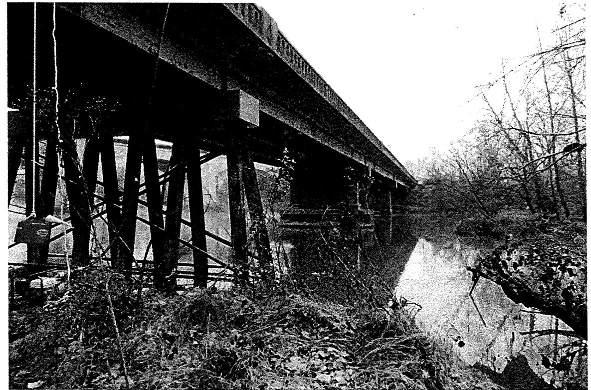
Looking down station.
