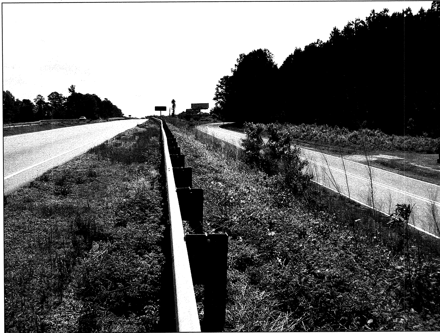
LOOKING EAST (UPSTATION) TOWARD EXISTING BRIDGE ALONG WEST APPROACH FROM APPROXIMATE STATION 19+00.
