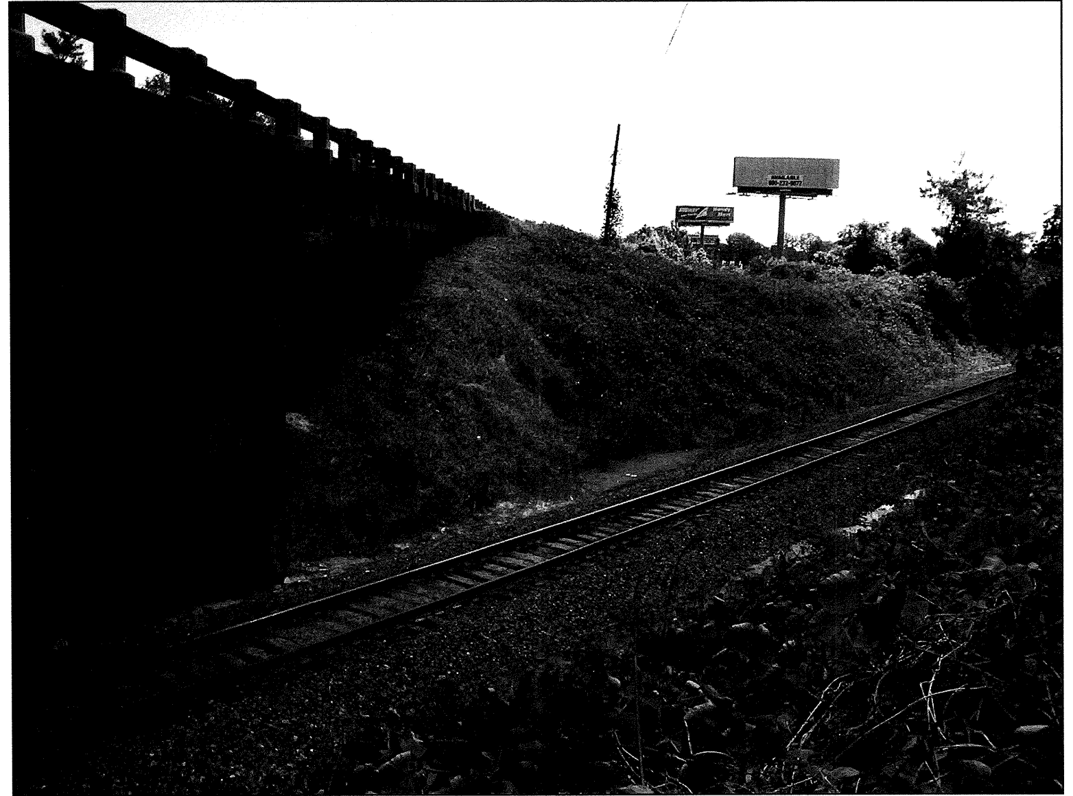
LOOKING EAST (UPSTATION) FROM RIGHT OF -L- ALONG EXISTING BRIDGE .
