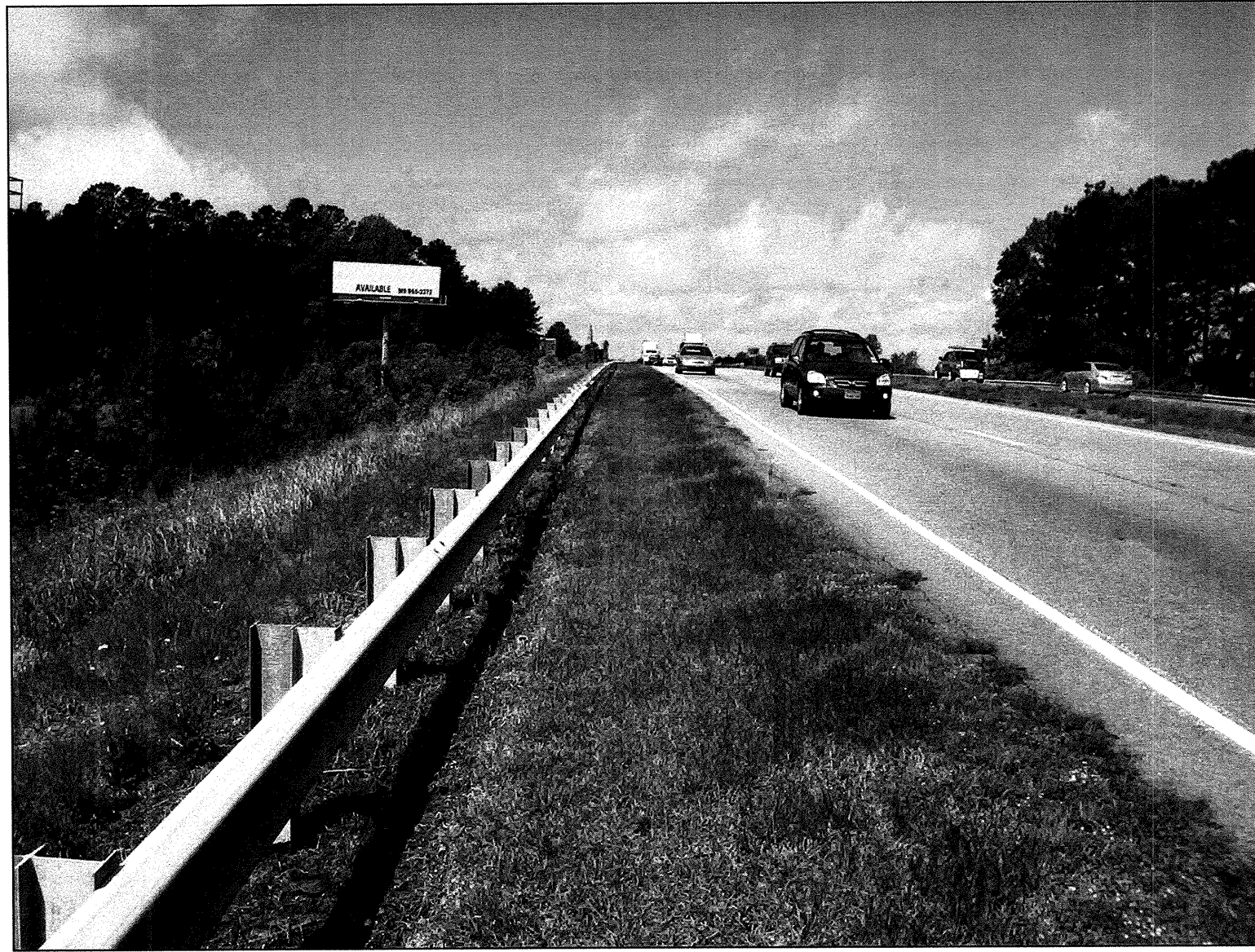
LOOKING WEST (DOWNSTATION) TOWARD EXTISING BRIDGE ALONG EAST APPROACH FROM APPROXIMATE STATION 31+00.
