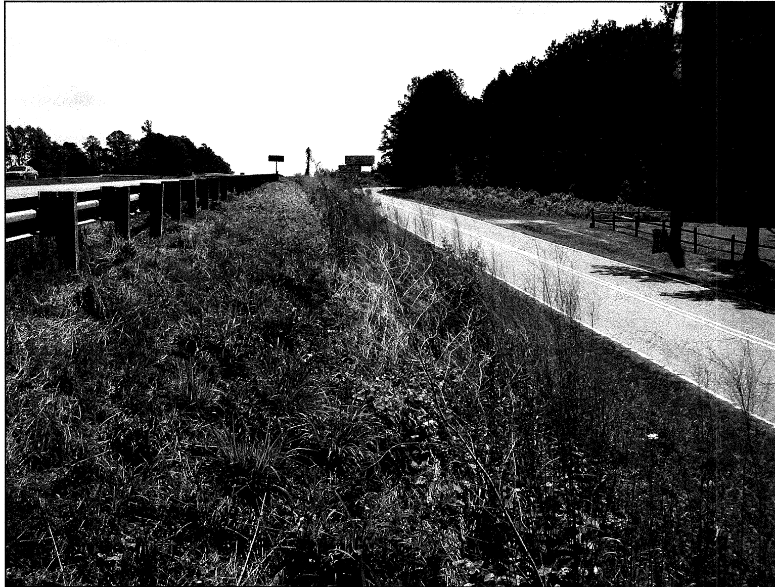
LOOKING EAST (UPSTATION) ALONG -WL- FROM BEGINNING OF WALL, APPROXIMATE STATION 19+75
