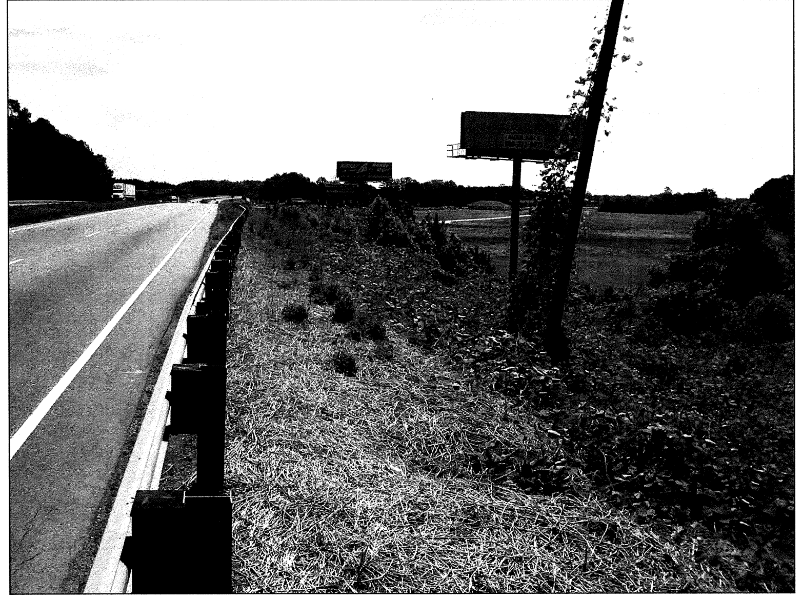
LOOKING EAST (UPSTATION) FROM WEST END OF BRIDGE, APPROXIMATE STATION 29+00.
