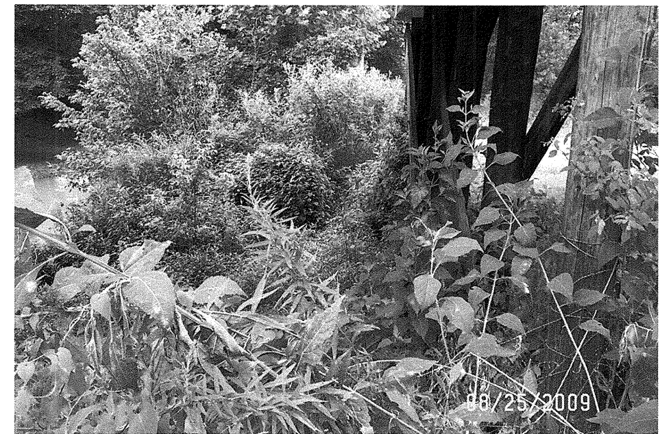
Photograph 4 – View Right to Left Across Bent-2
