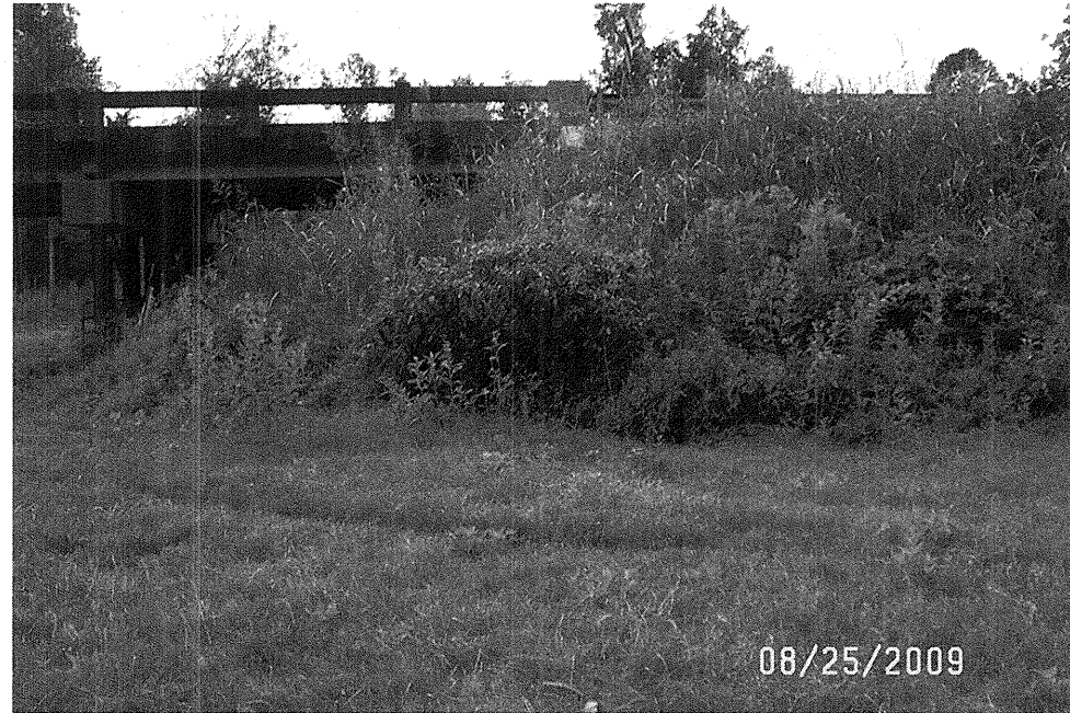
Photograph 1 – View Left to Right Across End Bent-1
