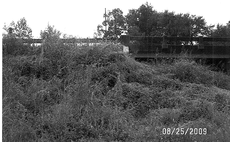
Photograph 6 – View Left to Right Across End Bent-2
