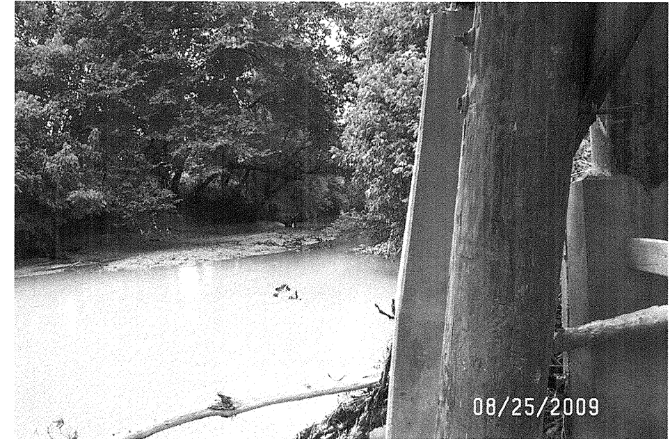
Photograph 7 – View Upstream from Centerline on West Side of Creek
