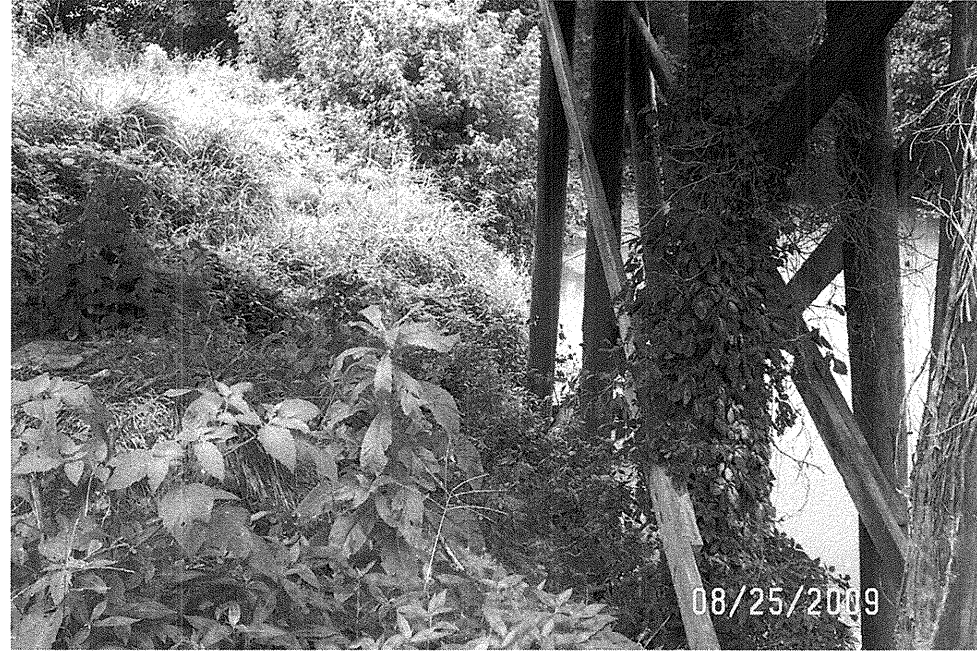
Photograph 5 – View Left to Right Across Bent-3
