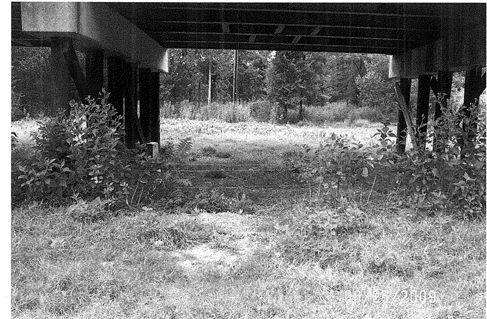
Photograph 3 – View Left to Right Across Bent-1
