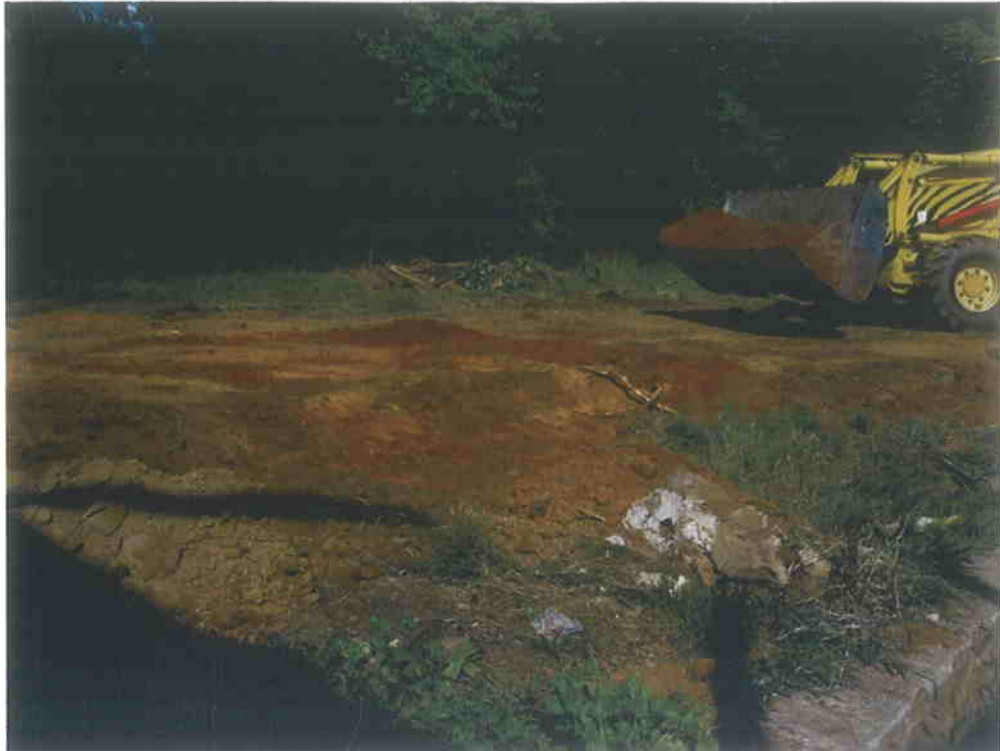
Photograph 5: View of grading of UST excavation at Parcel 9, 121 Hibriten Drive.
