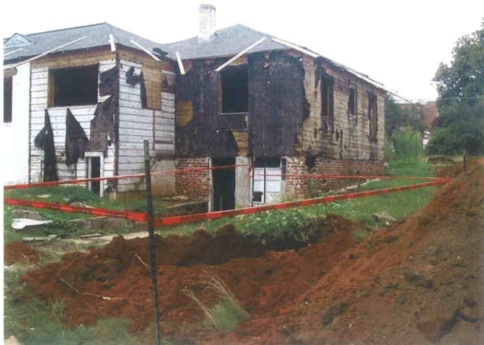
Photograph 4: View of over-excavation and stock-piled soil at Parcel 9, 121 Hibriten Drive.
