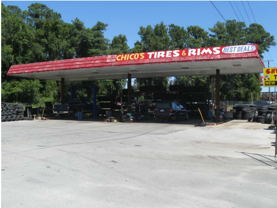
Parcel 905 – Louise Crumbley Property, looking east
