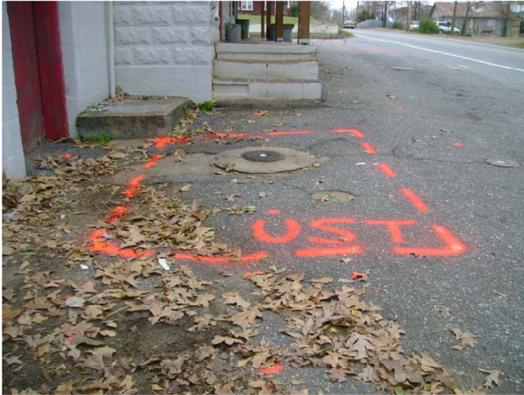
Parcel 53 – Howard & Rebecca Mull Property, looking north. Photo shows approximate marked location of probable UST No. 1 near the southeastern building corner.
