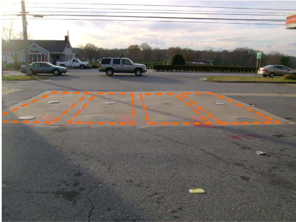
Parcel 34 – KHT & H, LLC Property, looking west. Photo shows approximate marked location of four known UST's near the southwestern corner of the building.
