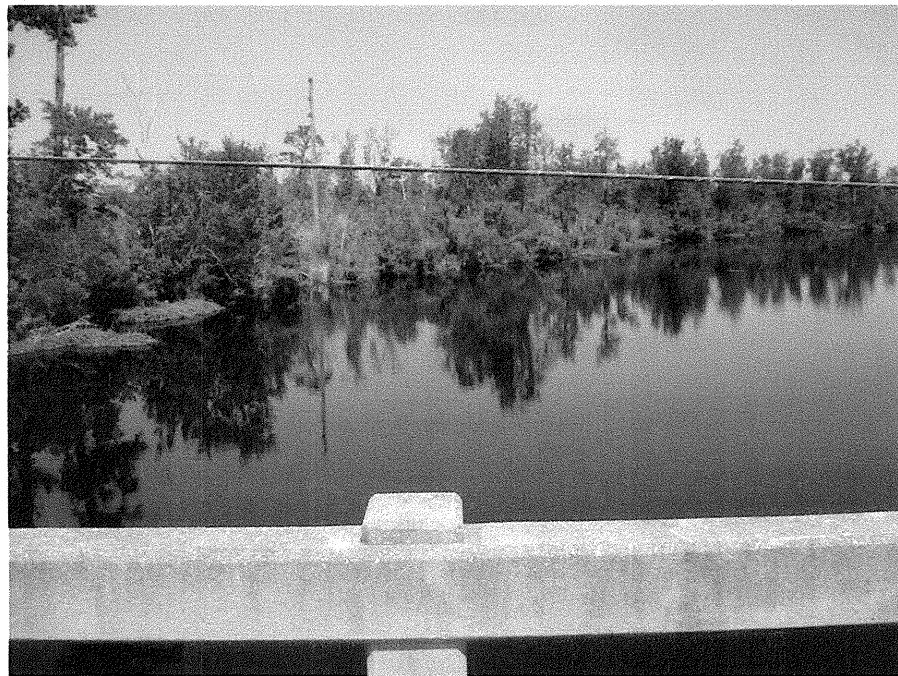
Photograph No. 6: This photograph was taken from the right side of the -L- alignment, looking west, across proposed Interior Bent No. 3.
