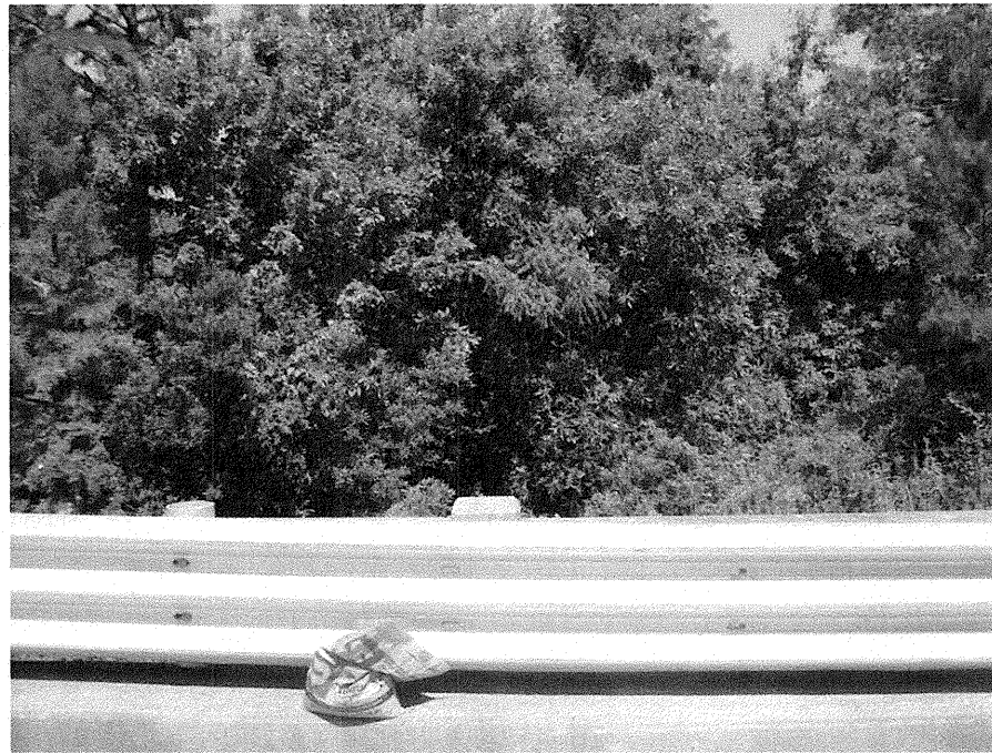
Photograph No. 13: This photograph was taken from the right side of the -L- alignment, looking west, across proposed End Bent No. 2.
