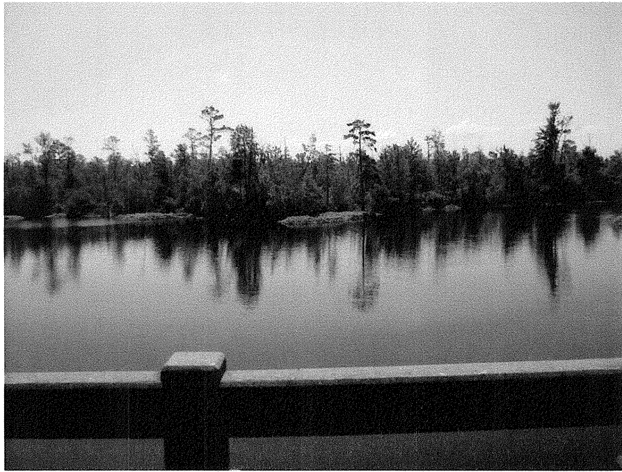
Photograph No. 9: This photograph was taken from the right side of the -L- alignment, from the center of the existing bridge deck, looking east (down river).
