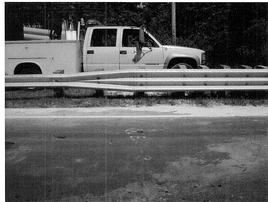
Photograph No. 3: This photograph was taken from the right side of the -L- alignment, looking west, across proposed End Bent No. 1.
