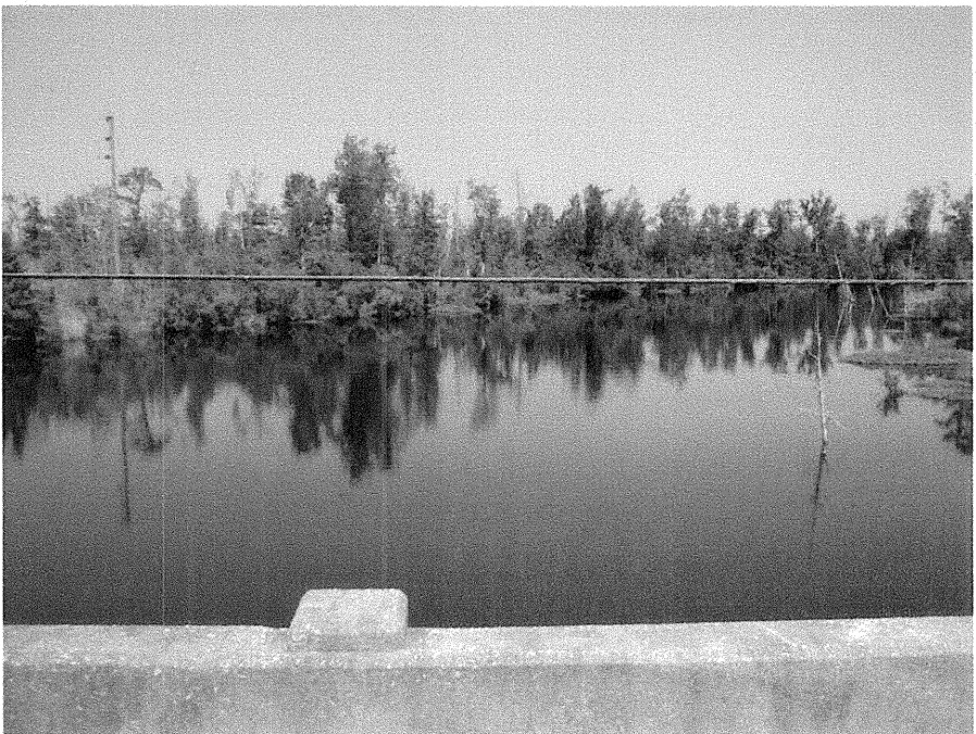
Photograph No. 7: This photograph was taken from the right side of the -L- alignment, looking west, across proposed Interior Bent No. 4.
