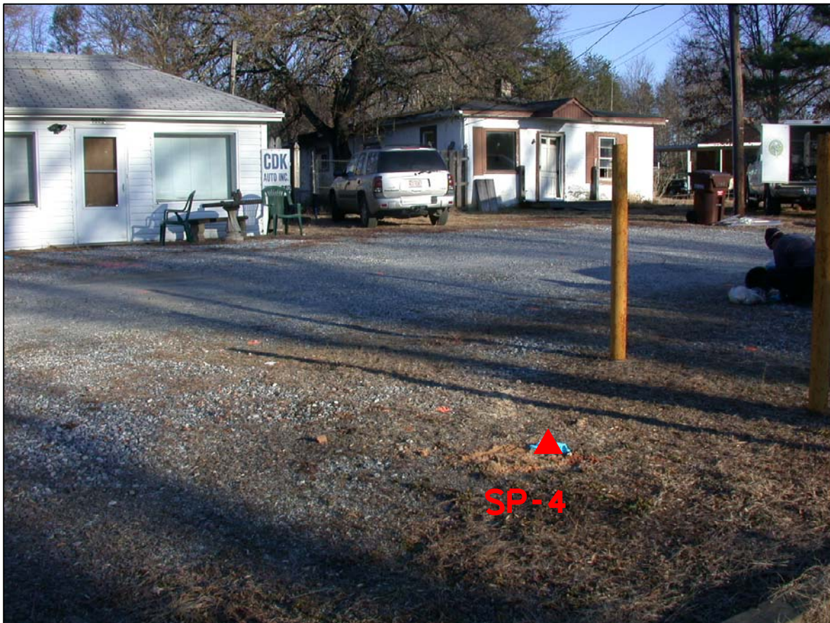
PHOTO 4 - BORING WITHIN PROPOSED R/W LOOKING SOUTHEAST
