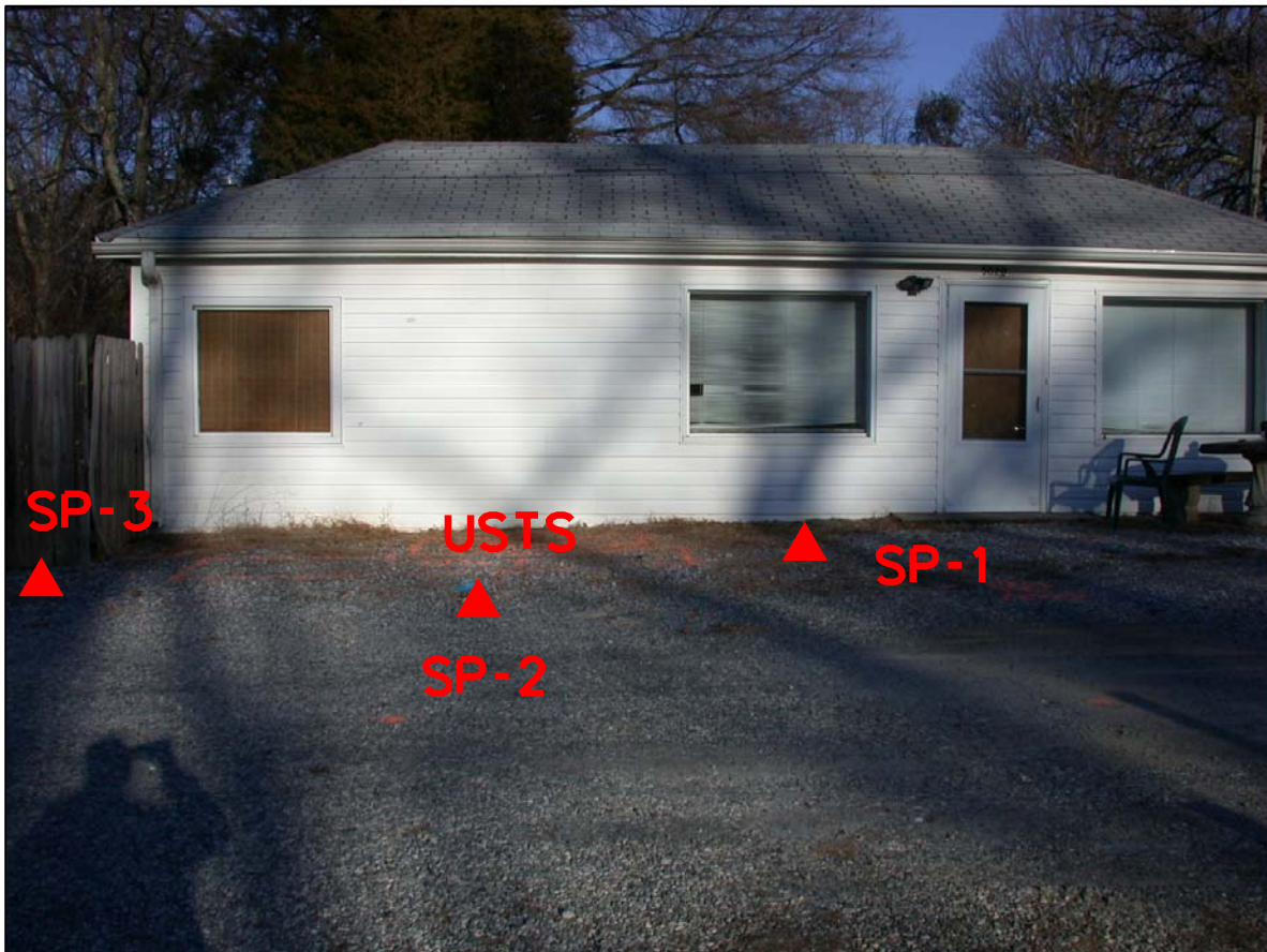
PHOTO 2 - BORINGS AT PROBABLE USTS LOOKING EAST
