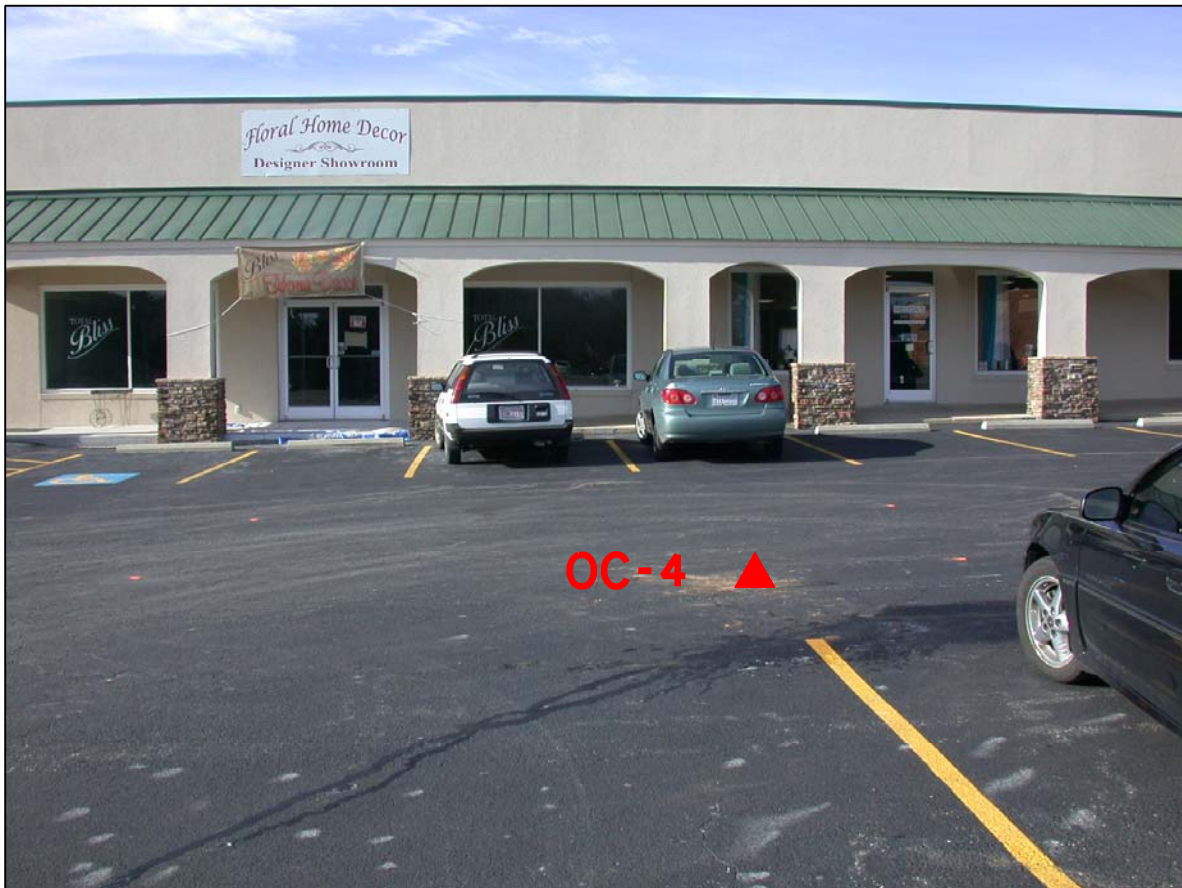
PHOTO 4 - BORING WITHIN PROPOSED R/W LOOKING WEST
