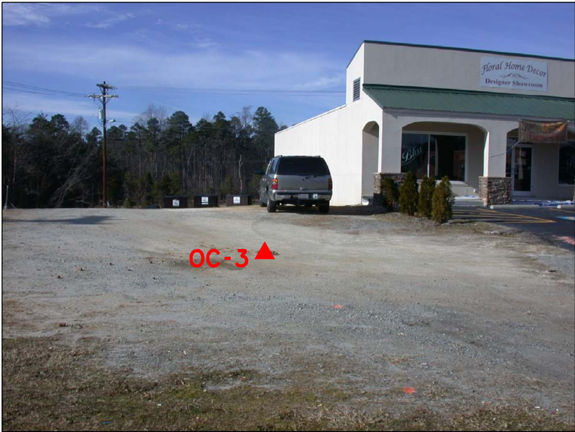
PHOTO 3 - BORING WITHIN PROPOSED R/W LOOKING WEST
