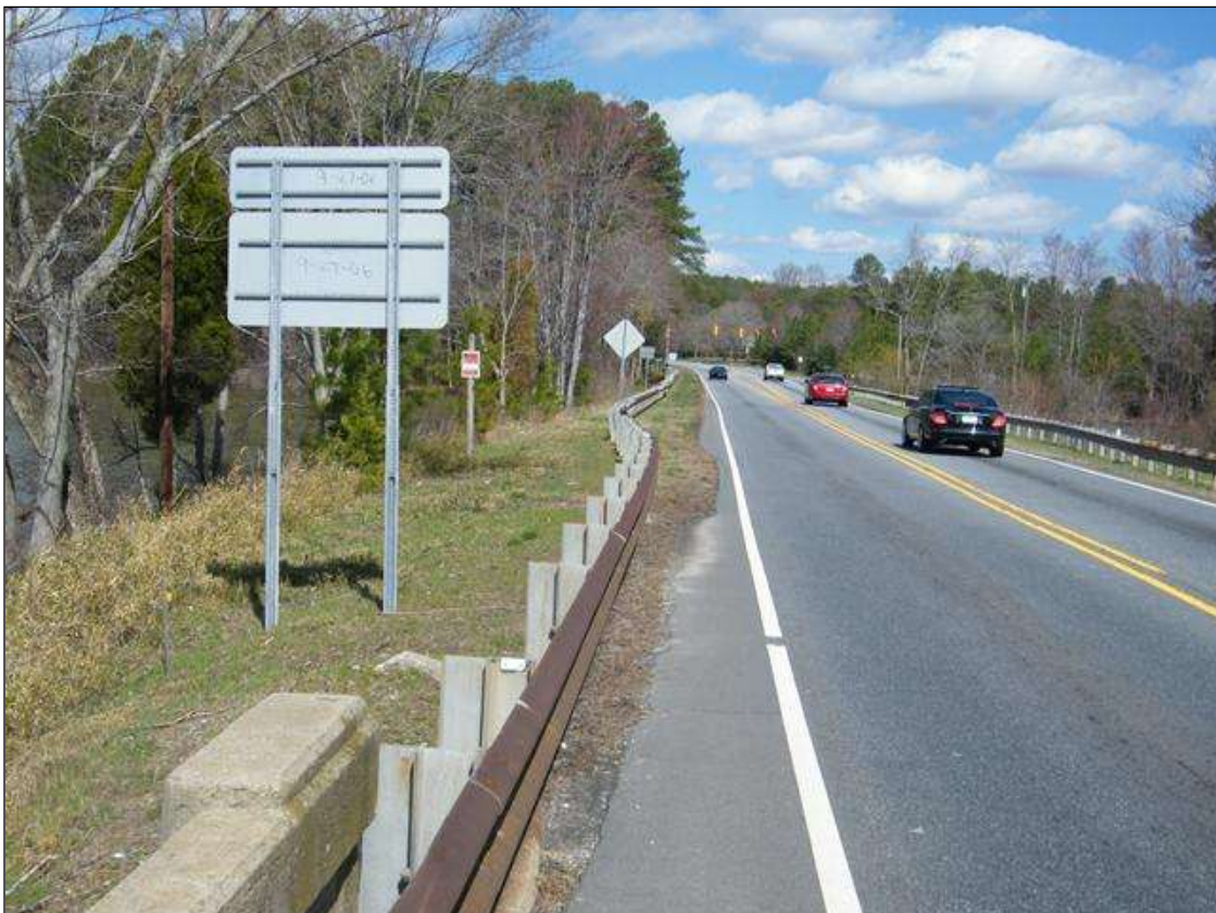
GUARDRAIL LOOKING NORTH
