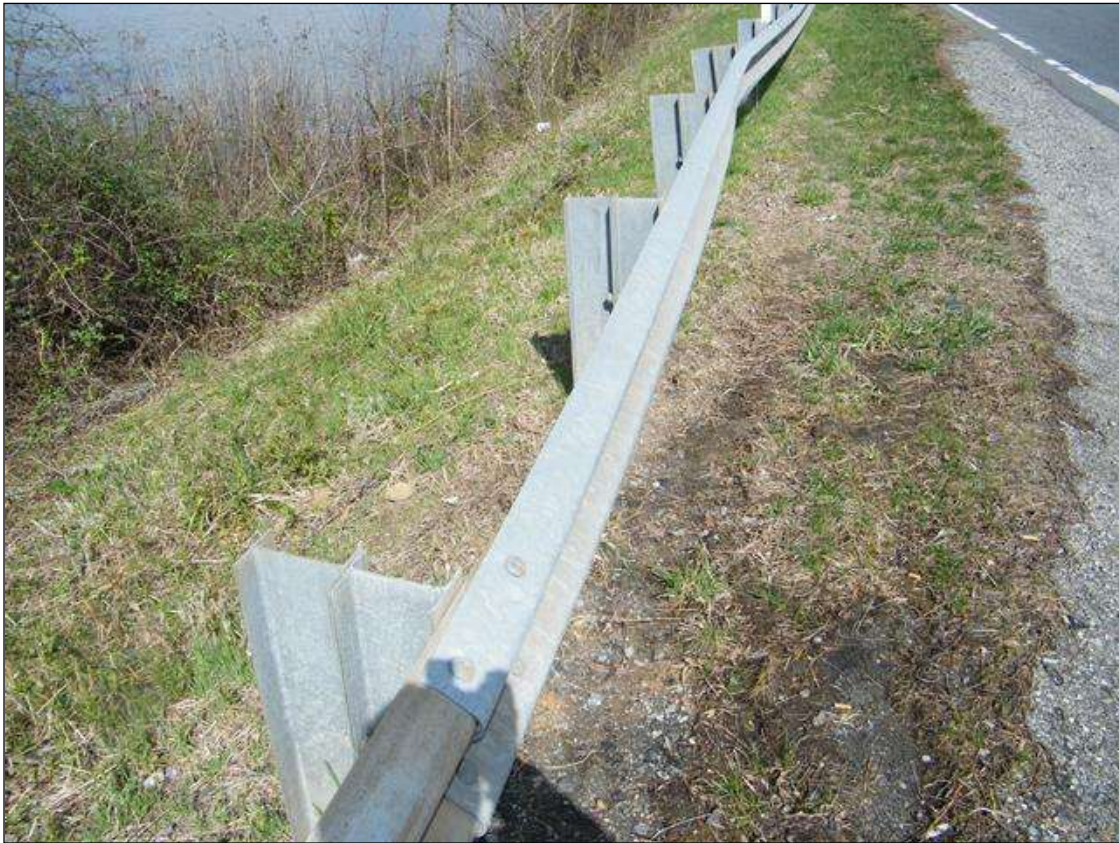
GUARDRAIL SPACING MIDWAY
