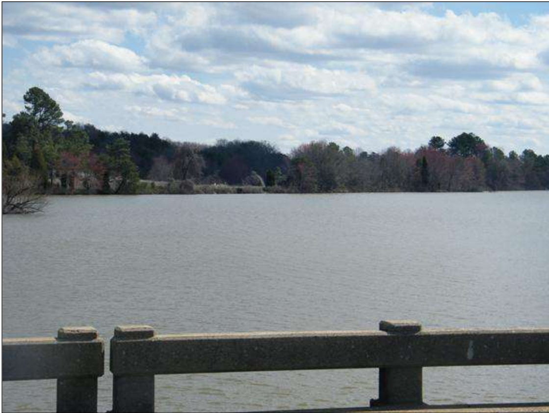
LOOKING EAST DOWNSTREAM FROM TOP
