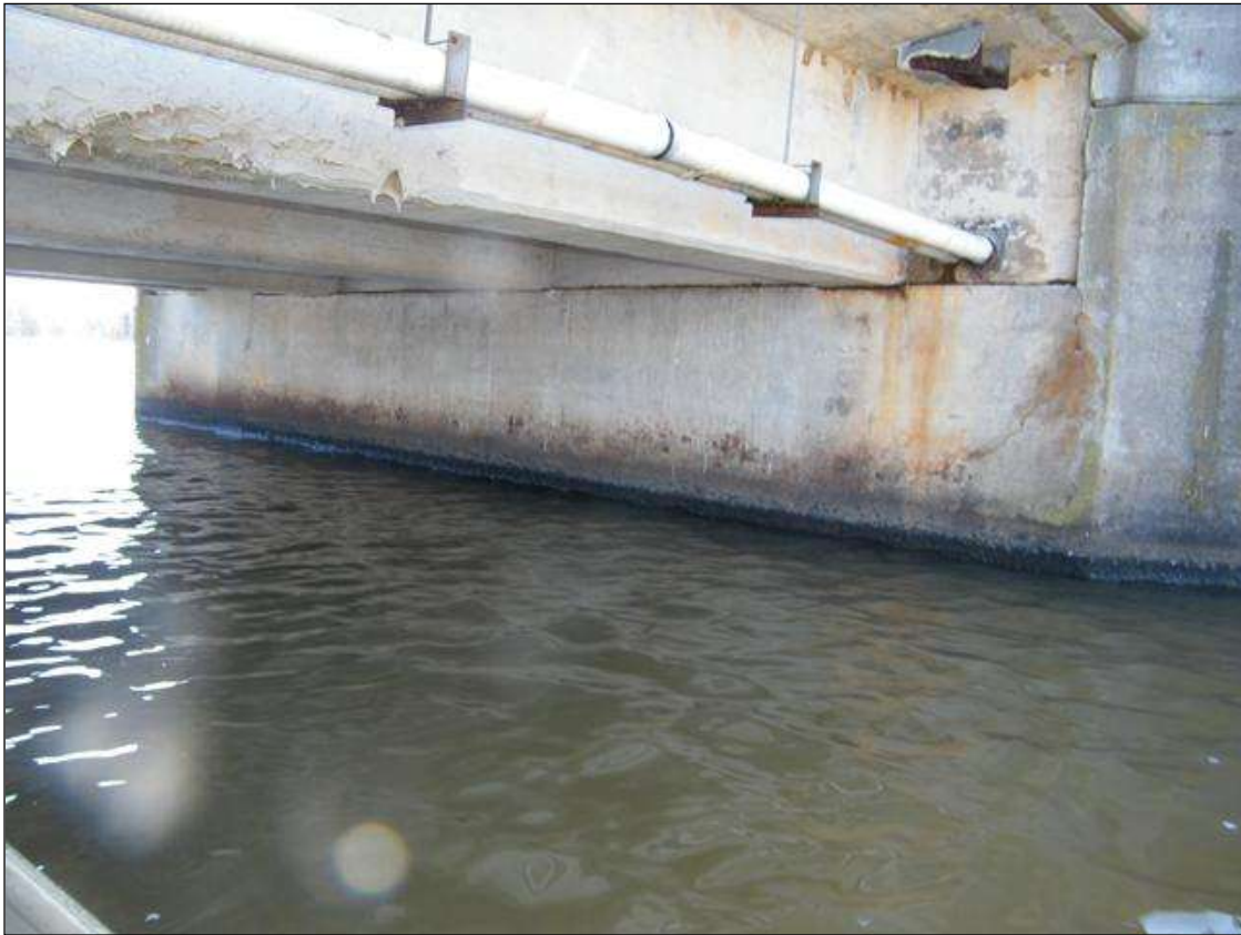
ABUTMENT 1, ABUTMENT 2 SIMILIAR
