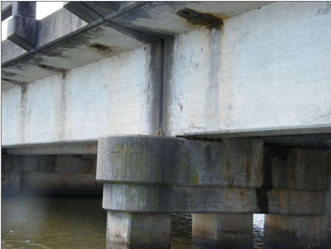
BEAM AT END OF CAP
