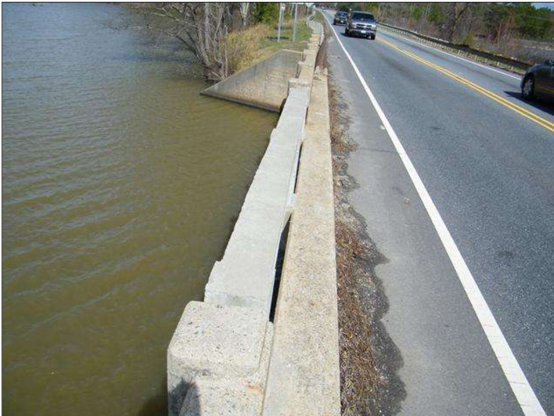
LEFT RAIL HAS BEEN REPAIRED IN SPAN 3
