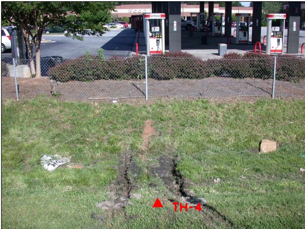
PHOTO 4 - BORING WITHIN PROPOSED R/W LOOKING EAST
