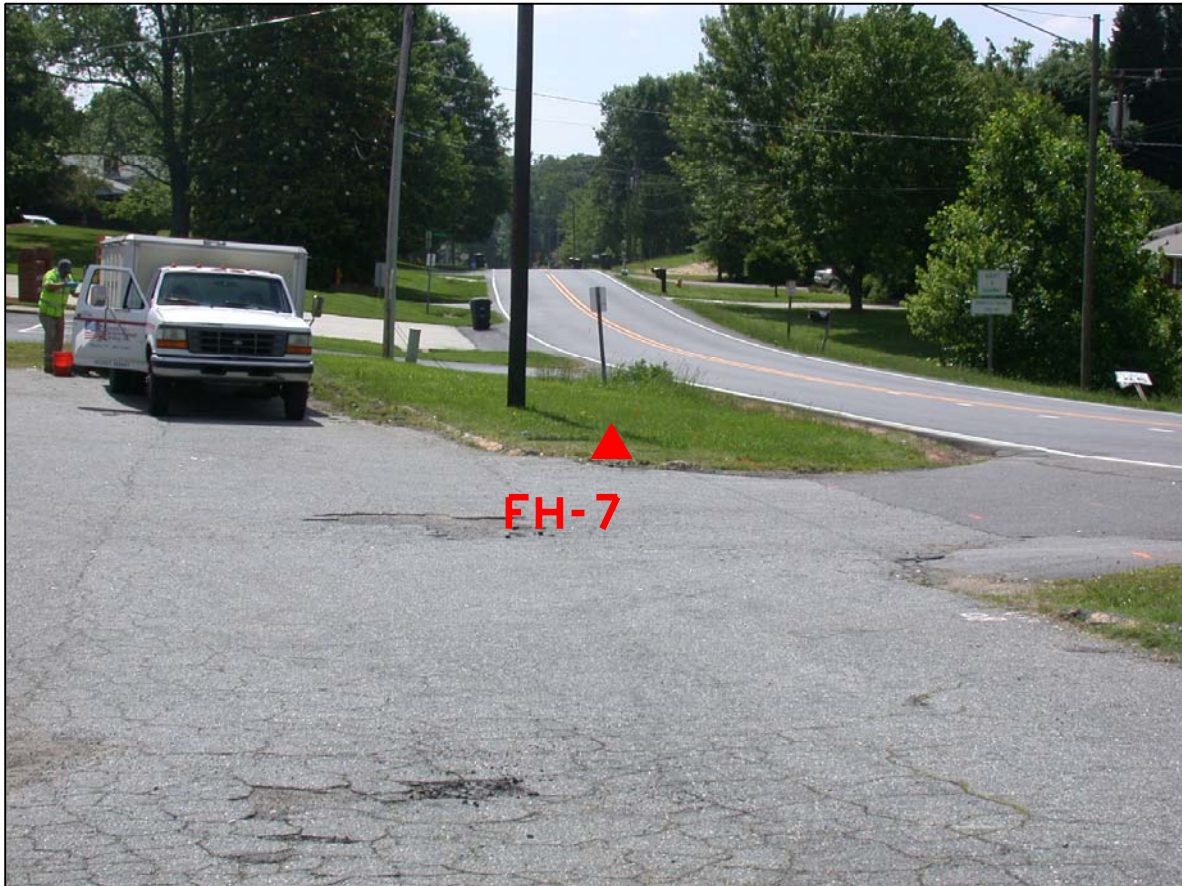
PHOTO 4 - BORING WITHIN PROPOSED R/W LOOKING EAST
