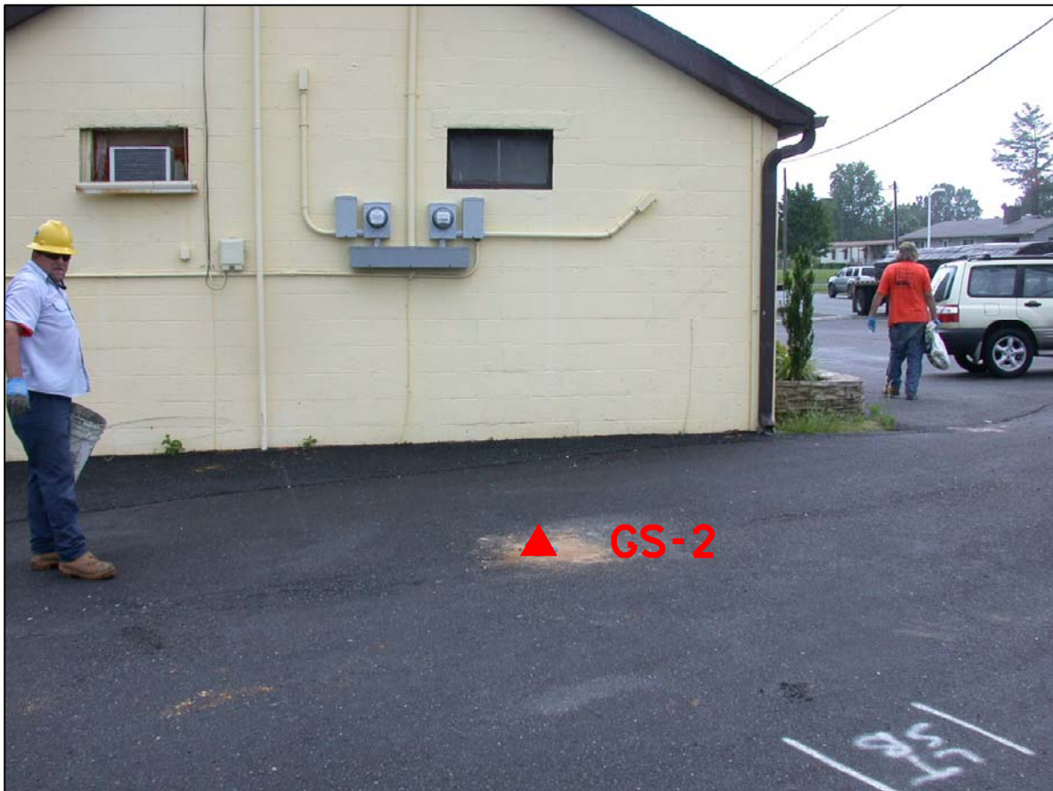
PHOTO 2 - BORING IN PROPOSED R/W LOOKING SOUTH
