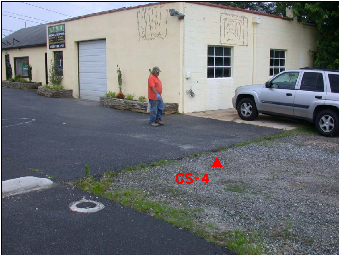
PHOTO 4 - BORING WITHIN PROPOSED R/W LOOKING NORTHEAST
