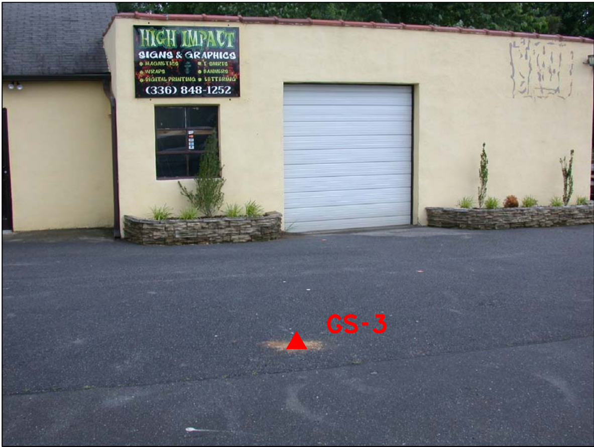
PHOTO 3 - BORING WITHIN PROPOSED R/W LOOKING EAST
