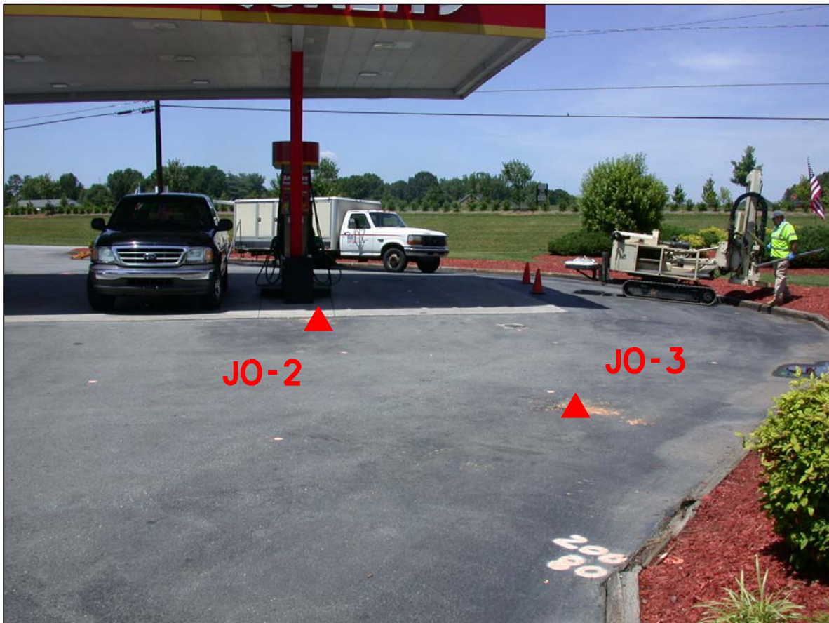
PHOTO 2 - BORINGS IN PROPOSED R/W LOOKING NORTH
