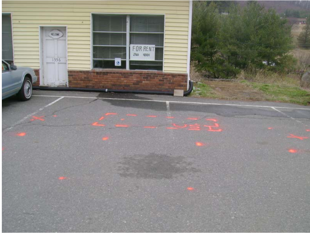
Parcel 7 – Talmadge S. Shepherd Property, looking northeast. Photo shows approximate marked location of the probable UST near the southwest corner of the southern building.
