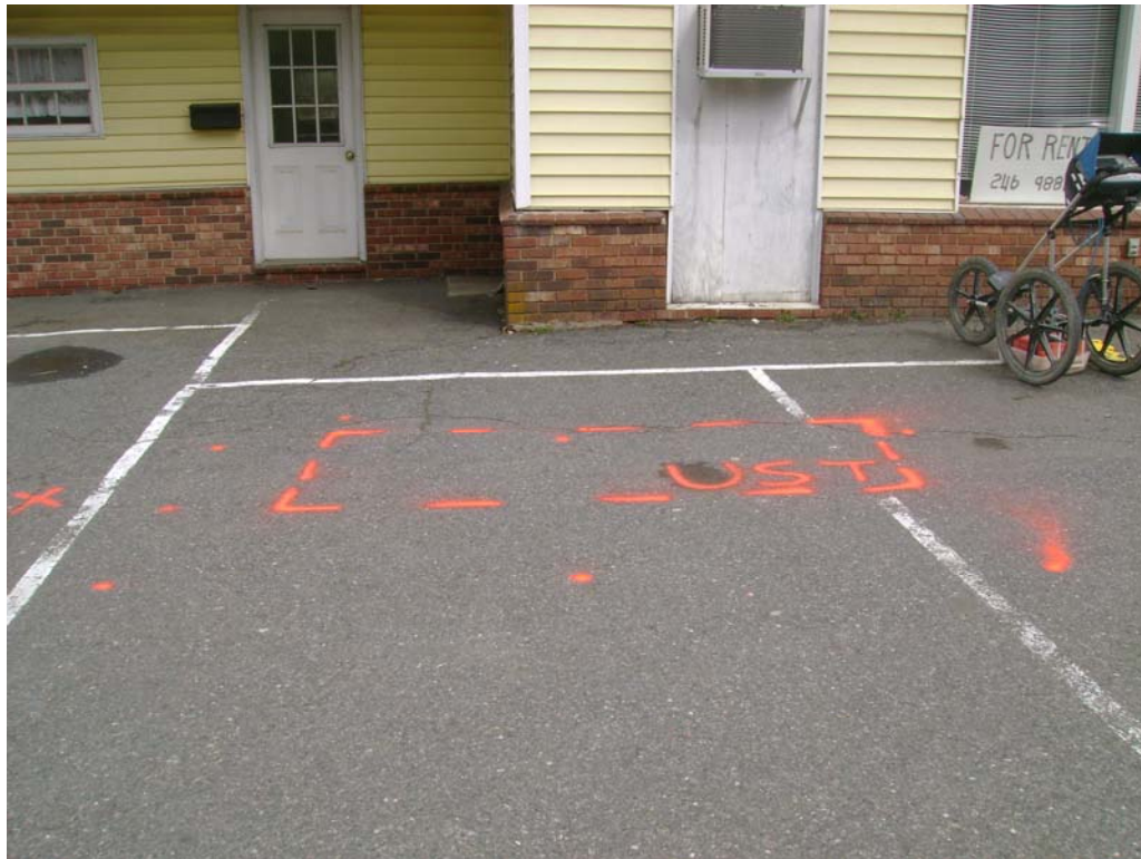
Parcel 7 – Talmadge S. Shepherd Property, looking northeast. Photo shows approximate marked location of the probable UST near the middle of the front side of the southern building.
