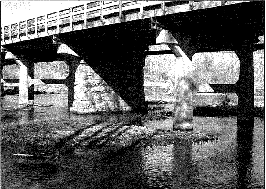
VIEW OF TYPICAL STONE MASONRY SUPPORT
