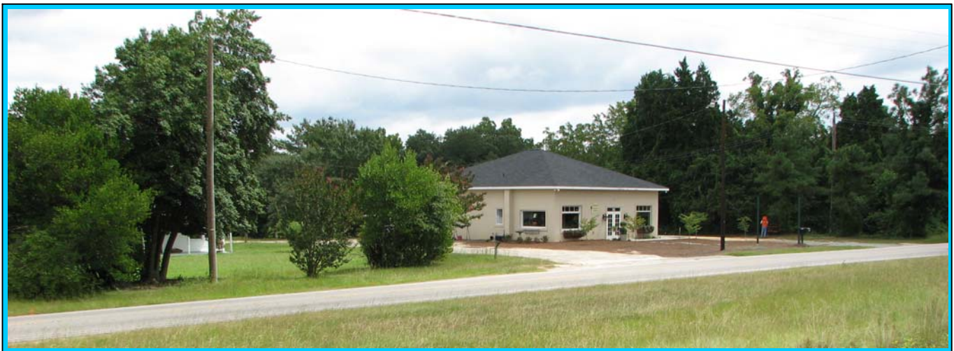
The photograph shows the Right-of-Way portion of the Fulcher property (Parcel 7). The photograph is viewed in an easterly direction.
