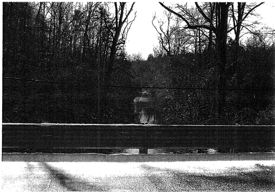
View Looking Downstream of Denson's Creek
