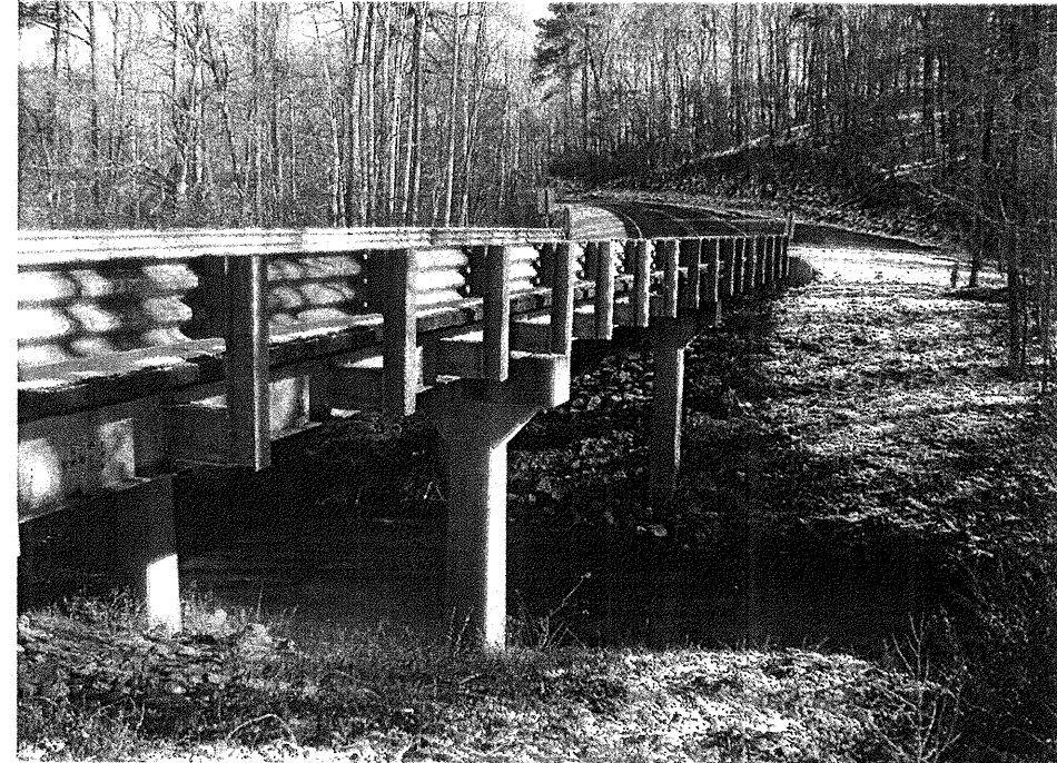
View of Bridge from Downstream side at existing End Bent 1
