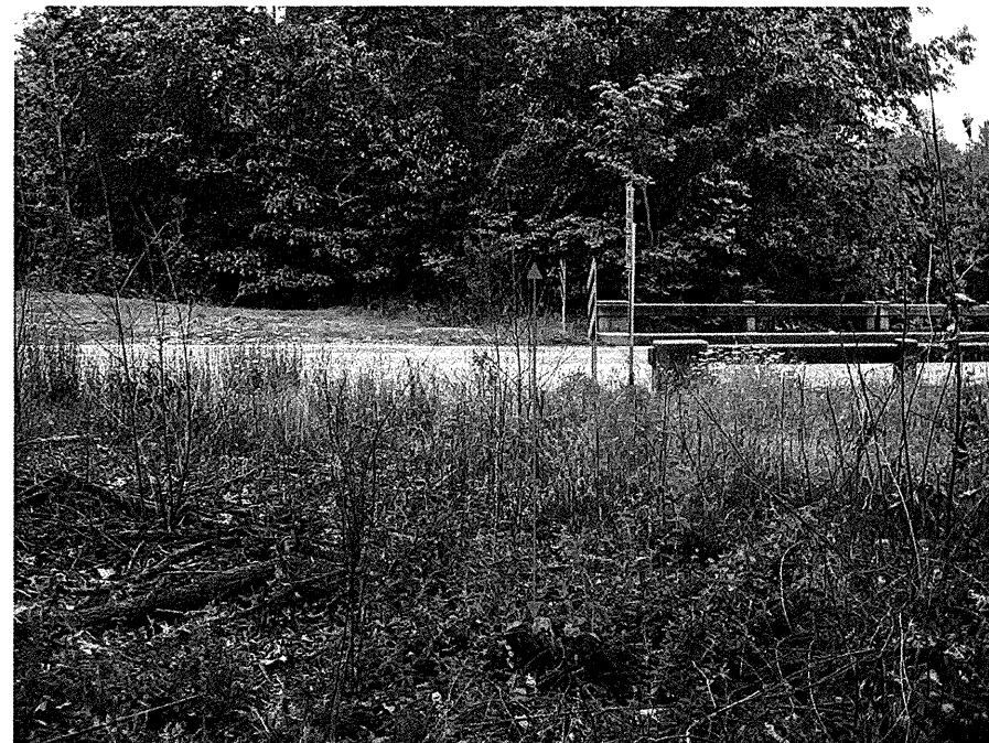
Photograph No. 2: View of End Bent 1 Section looking northeast.
