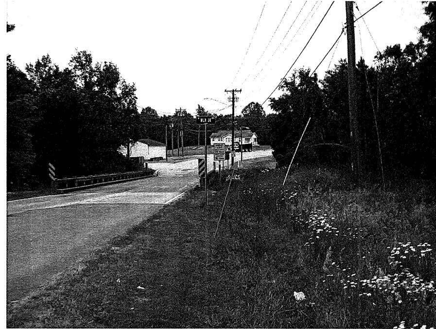
Photograph No. 1: View of Profile looking southeast.
