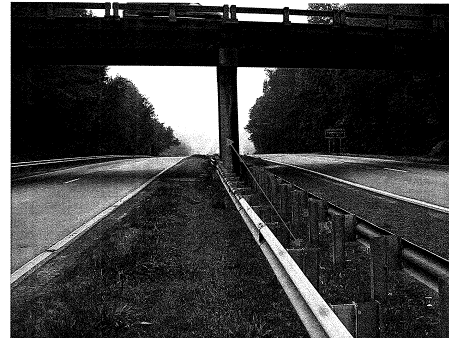
Photograph No. 3: View of Bent 1 Section looking northeast.
