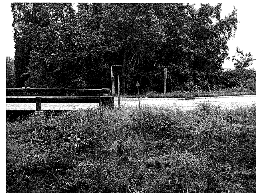
Photograph No. 4: View of End Bent 2 Section looking northeast.
