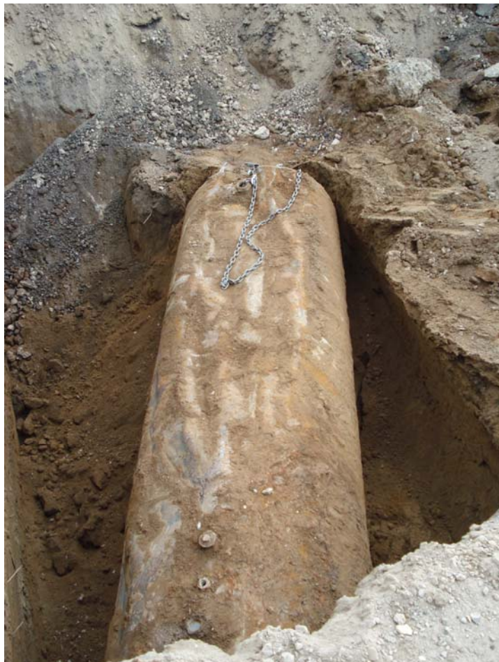
Photograph 2: View looking east at removal of UST #003.
