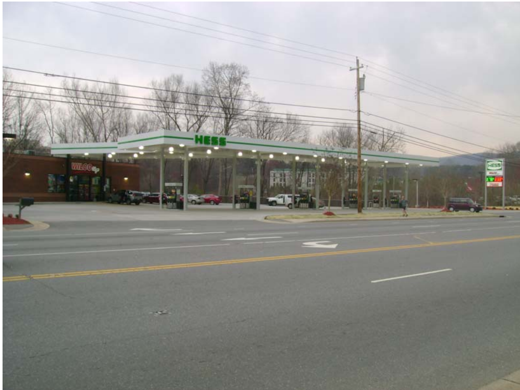
Parcel 2 – Jerry & Steve Issacs Property, looking northeast
