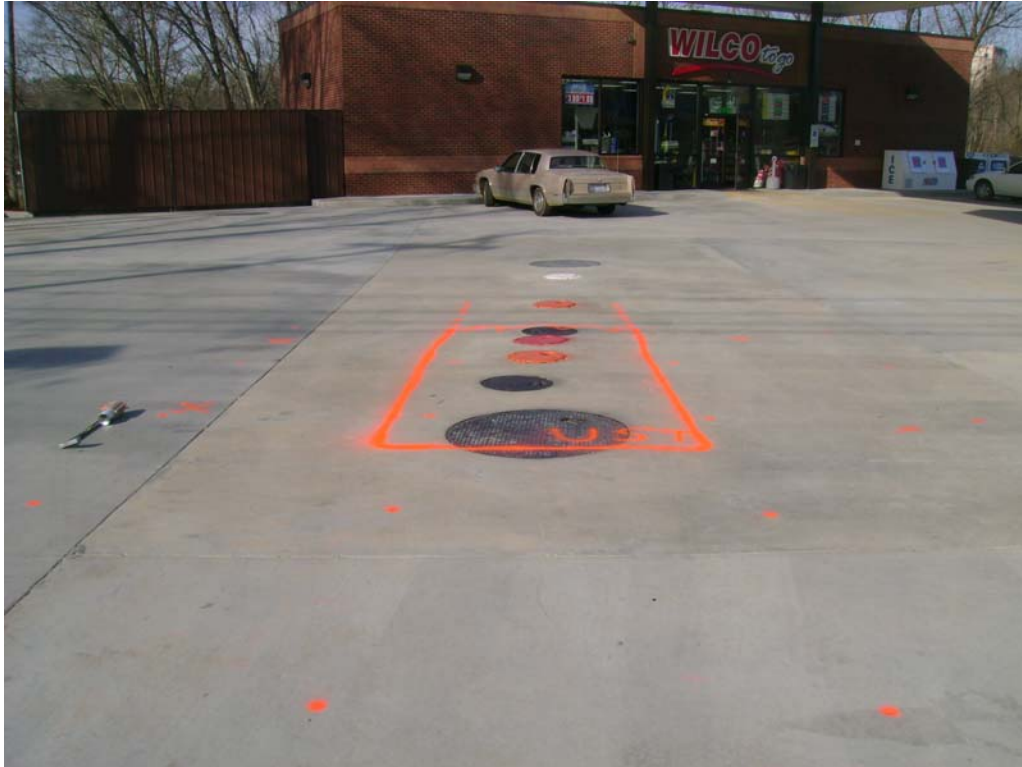
Parcel 2 – Jerry & Steve Issacs Property, looking northeast. Photo shows approximate marked location of the known UST near the westernmost corner of the canopy.
