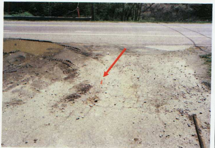
Photograph 6: Looking south at one of the proposed drainage piping locations (GP-10).
