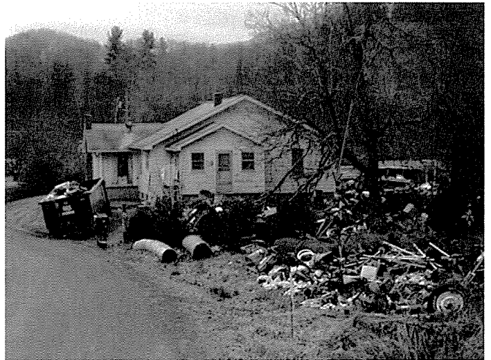
Photograph 4: Same view but closer.
