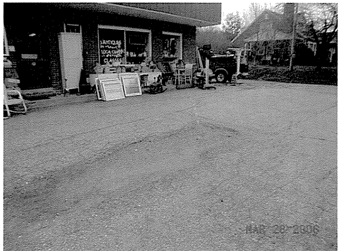
Photograph 4: Footprint of former pump dispenser island and remaining product line marked by orange paint.
