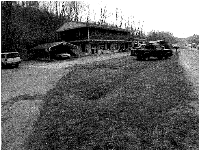
Photograph 3: Area of former gasoline USTs adjacent to eastern side of subject property building beneath car port.
