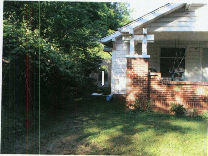
Photograph 1: View of subject property house. Note location of UST (Arrow).
