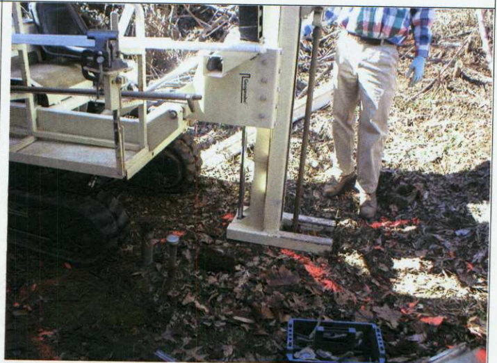
Photograph 6: View of drilling activities. This photo shows the "GP-2" location.
