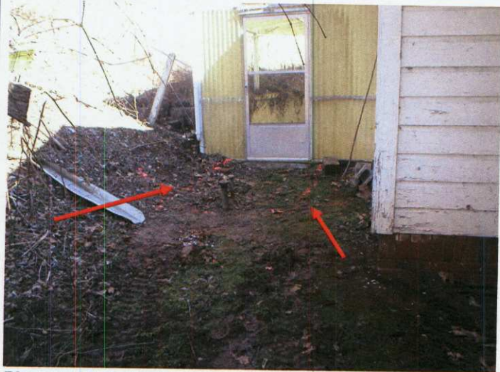
Photograph 3: Another view of UST. Orange markings note the boundary of the tank.
