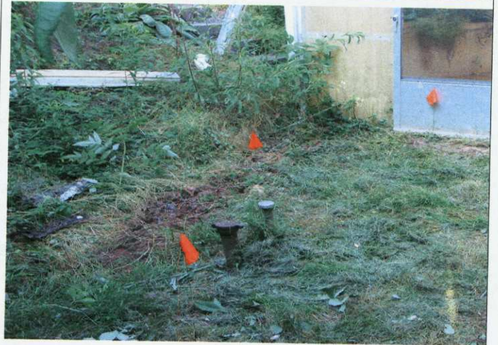
Photograph 2: Close-up view of heating oil UST. Flags outline the layout of the tank.
