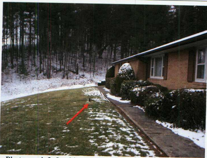
Photograph 3: Looking south. Note the fill port and vent pipe in the center of the photo.
