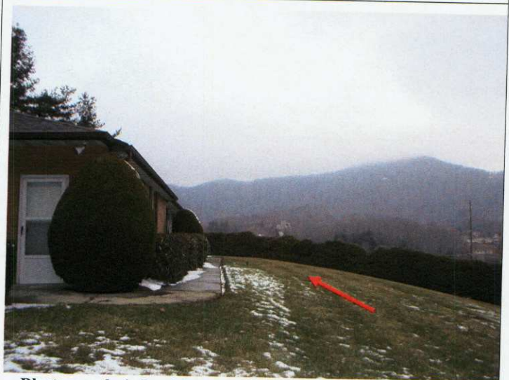
Photograph 4: Looking north. Note the fill port and vent pipe in the center of the photo.
