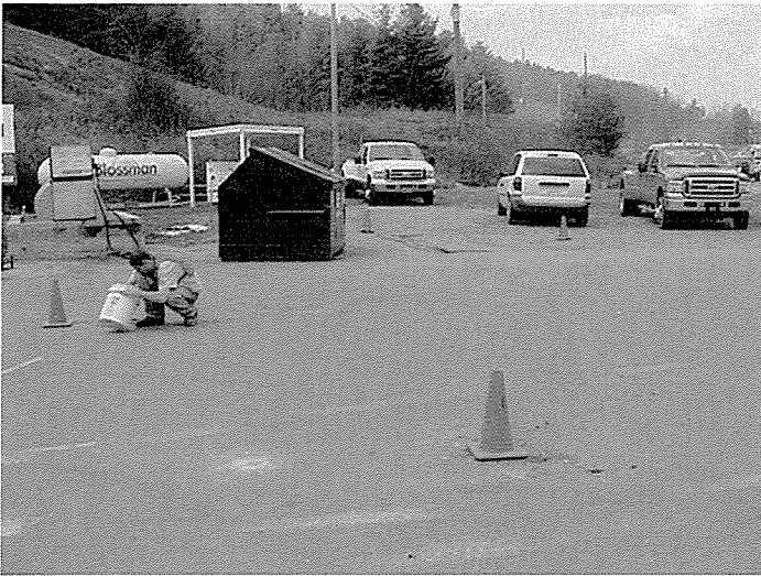
Borings GP1, GP12, GP5 and GP6 facing west
