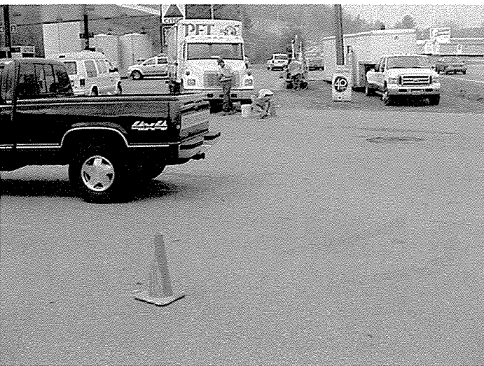
Boring GP9 and GP10 facing west
