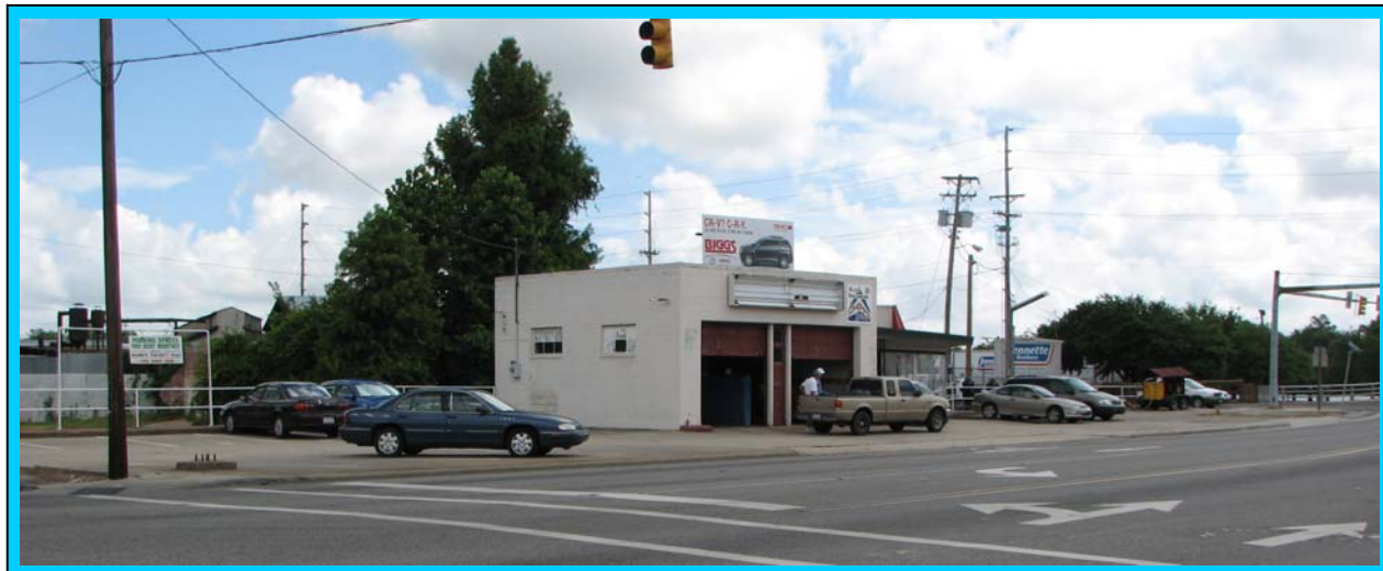
The photograph shows 610 East Elizabeth Street site (Mann Capital Properties, Limited) located at the intersection of East Elizabeth Street and North Water Street in Elizabeth City, North Carolina. The photograph is viewed in a northeasterly direction.
