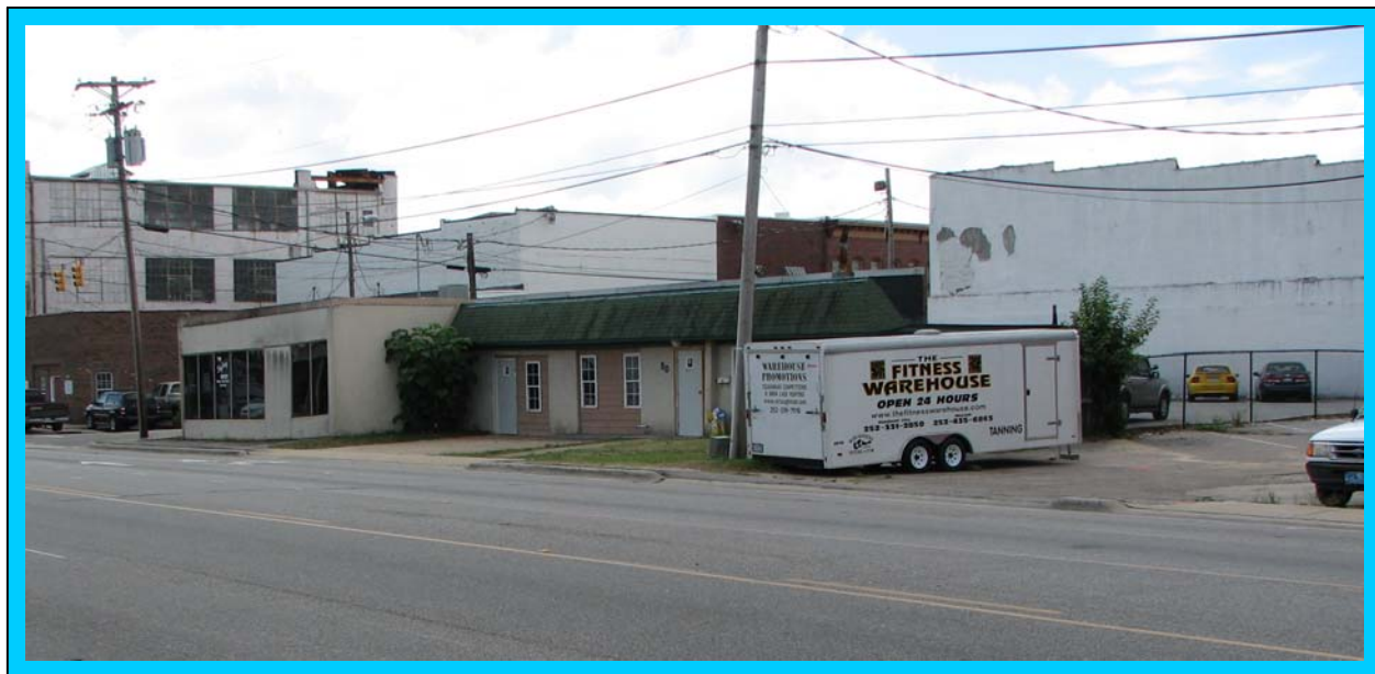
The photograph shows the 507 East Elizabeth Street site (Gracie Bernardo property, Parcel 15) located at the intersection of East Elizabeth Street and North Poindexter Street in Elizabeth City, North Carolina. The photograph is viewed in a southeasterly direction.
