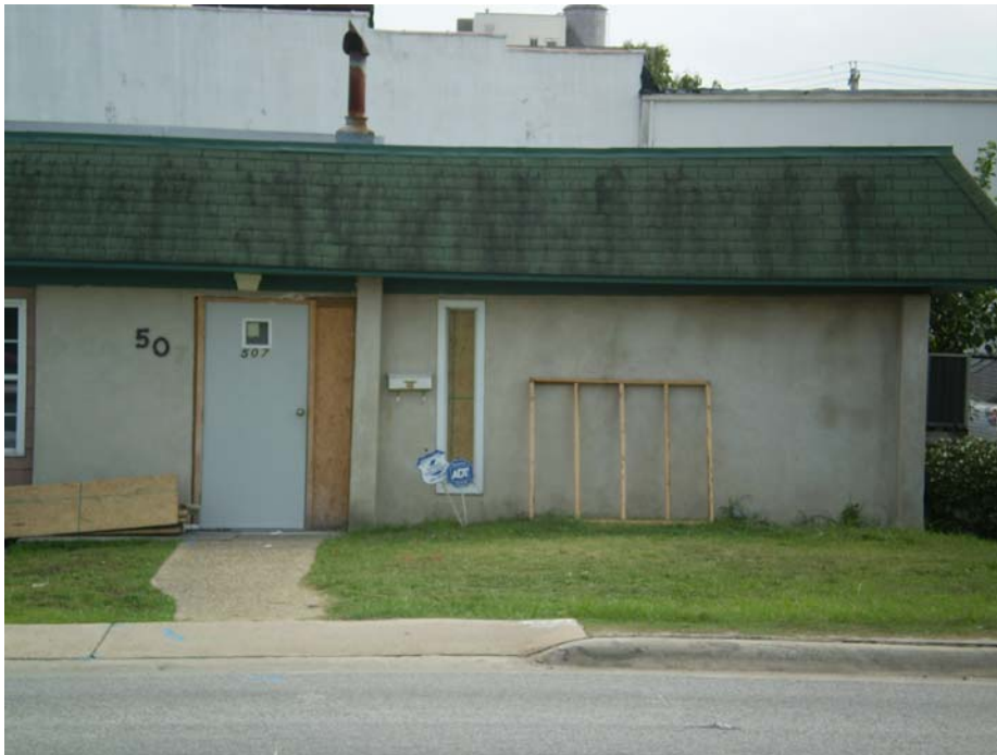
Photograph 2 – View of Parcel #15, looking south from East Elizabeth Street.
