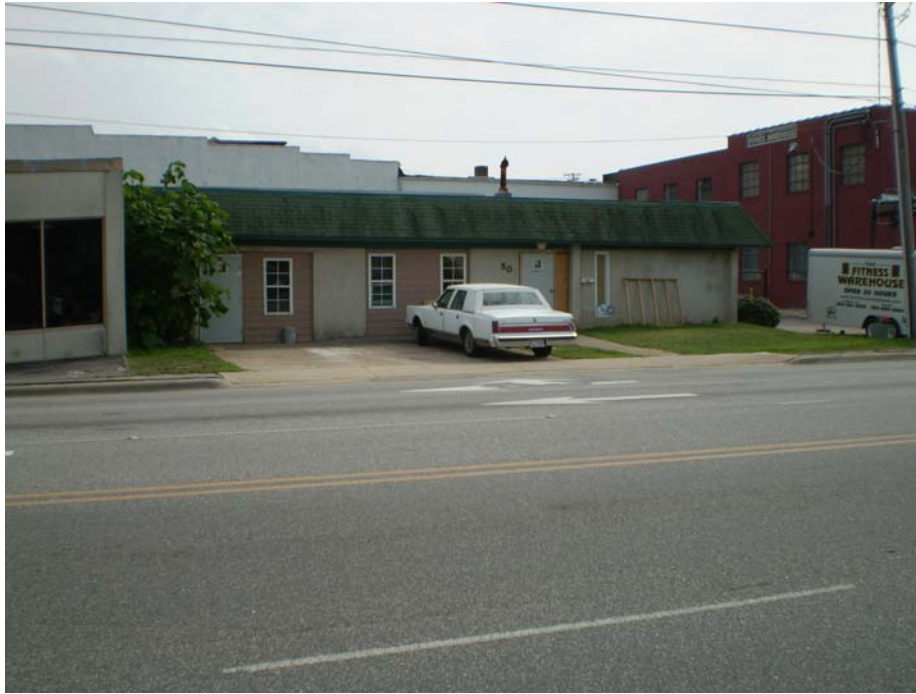
Photograph 1 – View of Parcel #15, looking south from East Elizabeth Street.
