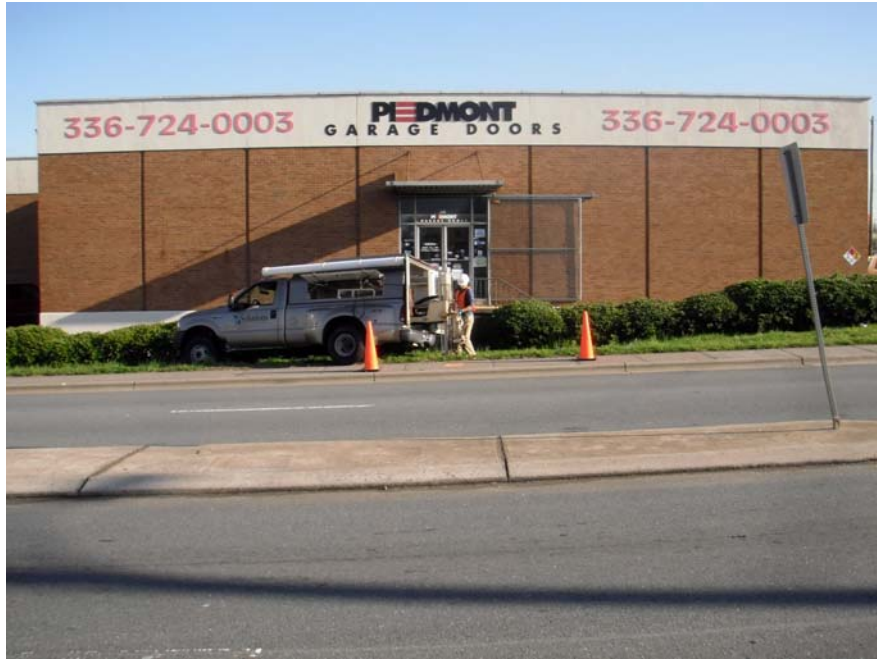
Photograph 1 – View of Parcel #2 store front, looking north from Martin Luther King Jr. Drive.
