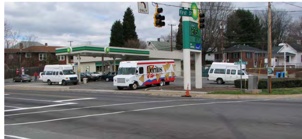
M. M. FOWLER PROPERTY - (PARCEL 29) BP GAS STATION/STORE 105 N. MARTIN LUTHER KING, JR. DRIVE
