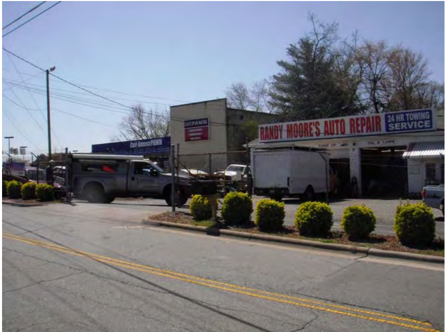
Photograph 1 – View of the Meryl B. Mabe Property looking southwest along Leo Street.
